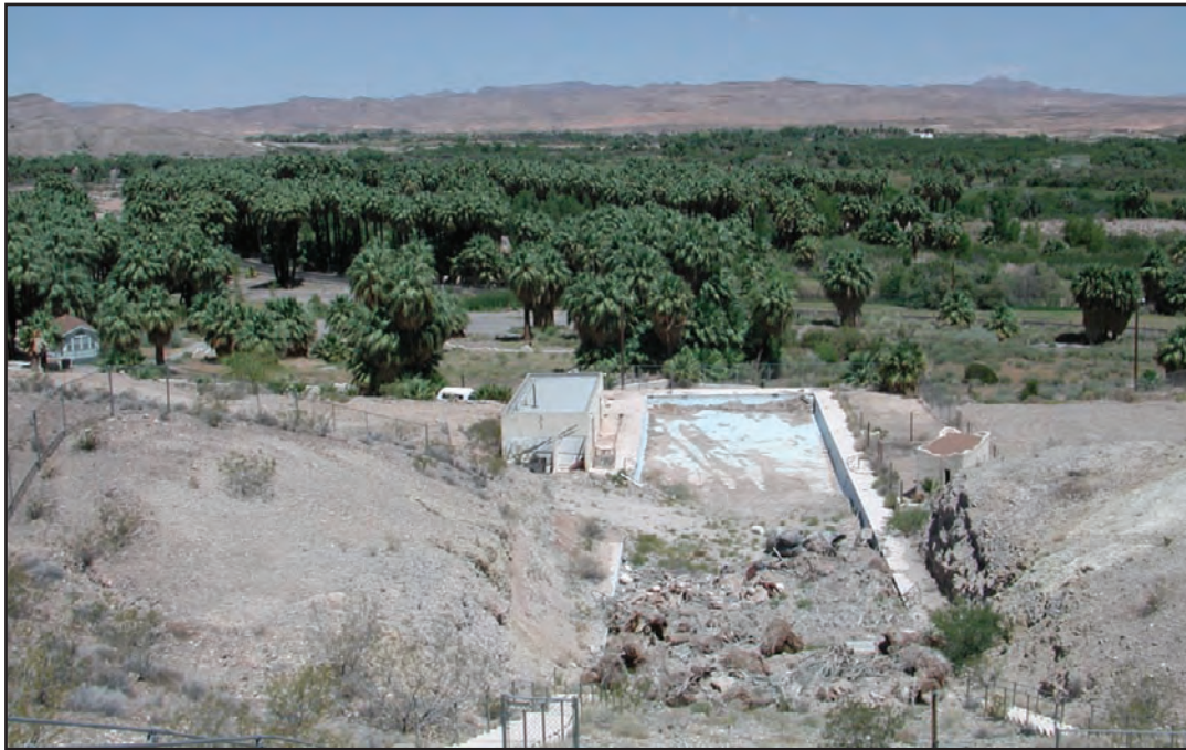
B. Remains of a water slide and pool.
