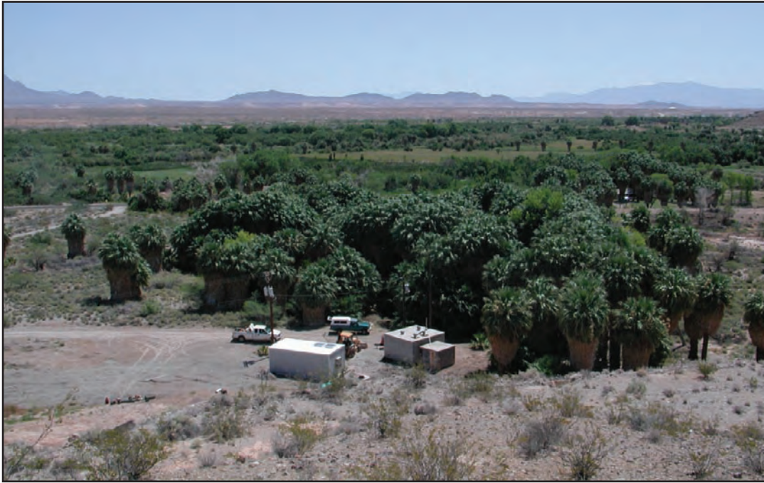
A. View of Moapa Valley Water District's old (right) and new (left) pump houses in the foreground.
