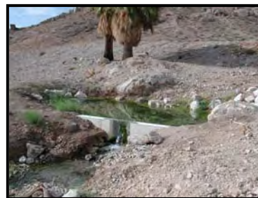
View of weir from downstream
