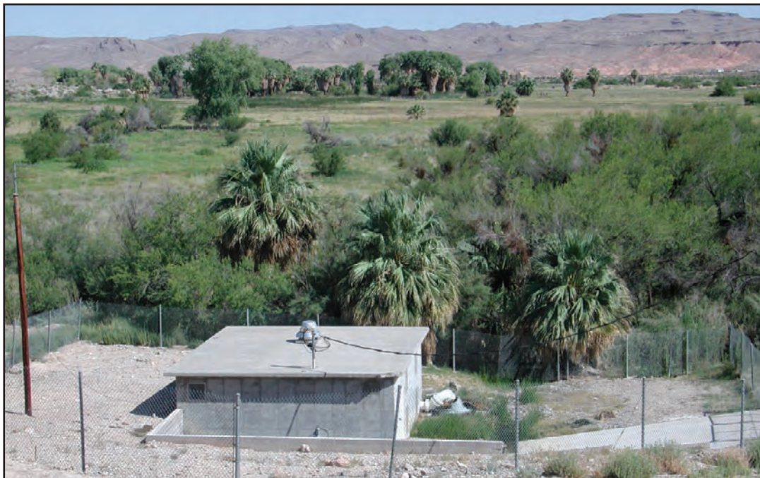
Figure A11. View of the Baldwin Springs area and the Moapa Valley Water District pump house in the Warm Springs area near Moapa, Nevada. Photographed in June 2004 by D. Beck.
