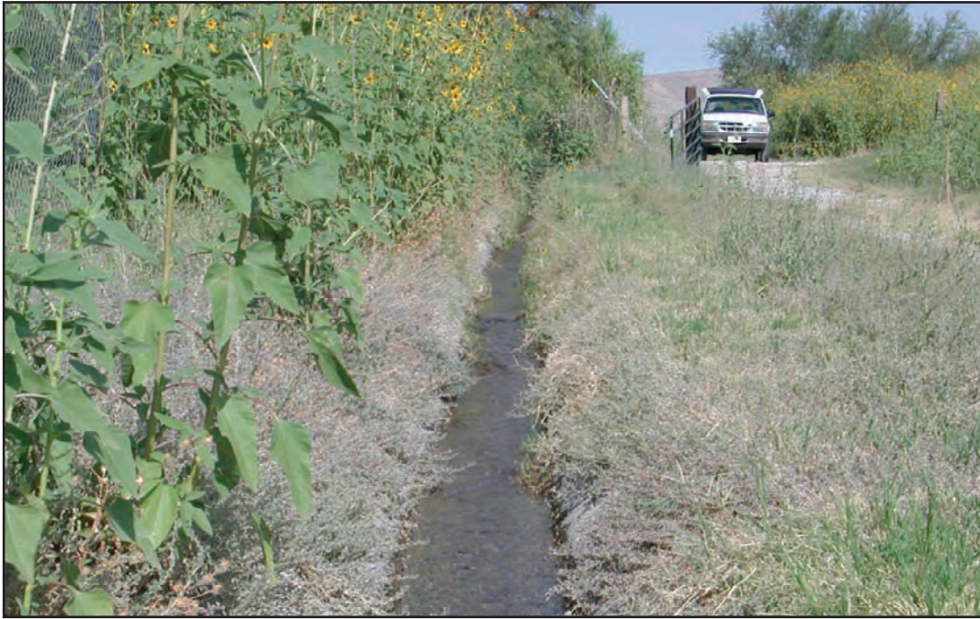
A. Concrete irrigation ditch east of Cardy Lamb Swimming Pond.
