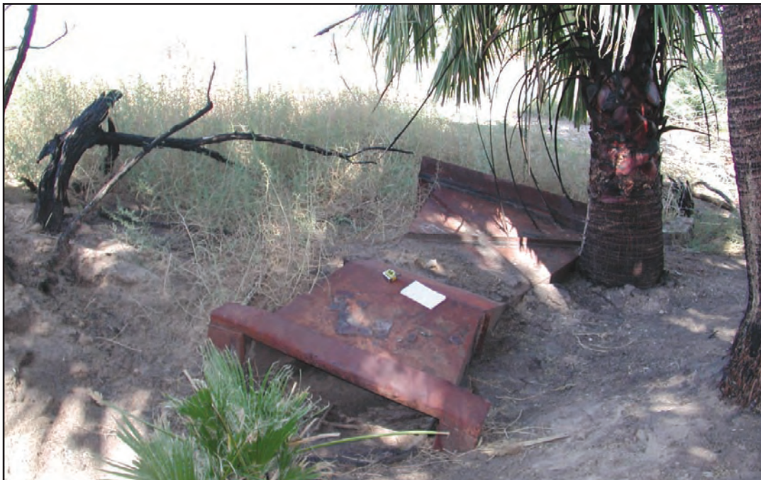
Figure B6. Former Big Wash flume on right bank of North Fork Muddy River in the Warm Springs area, near Moapa, Nevada. The flume is about 500 feet upstream of confluence with South Fork Muddy River. Photographed in September 2004 by D. Beck.
