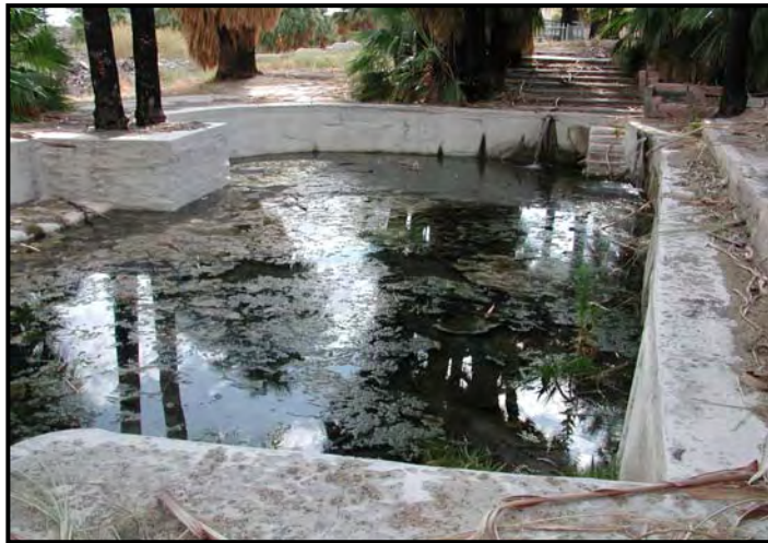
Swimming pool upstream of M-20
