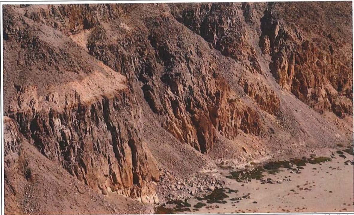
View along the northeast-southwest trace of the Maynard Lake Fault zone. Volcanic rocks highly fractured and faulted along fault zone. Maynard Lake (dry) in bottom of photograph.
