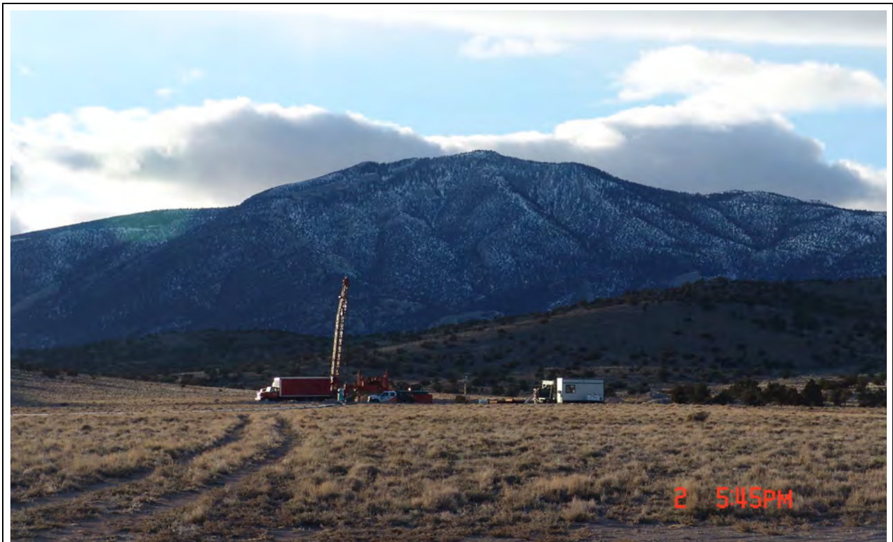
Figure A-1 184W105 Test Well Site, Facing Southwest
