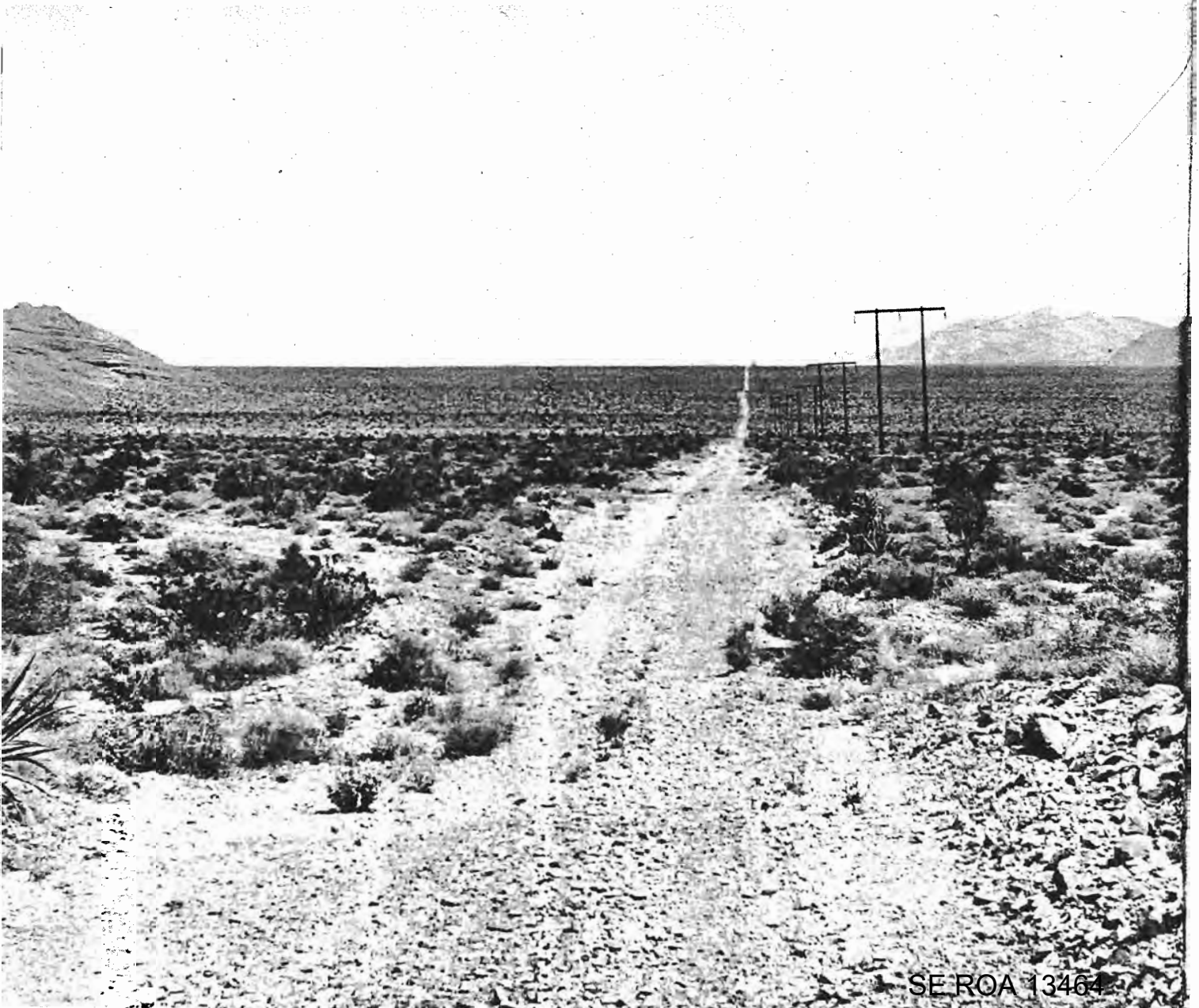
Caliente Power Line right-of-way forms southeastern boundary of proposed Las Vegas Range Wilderness Unit, at left.
