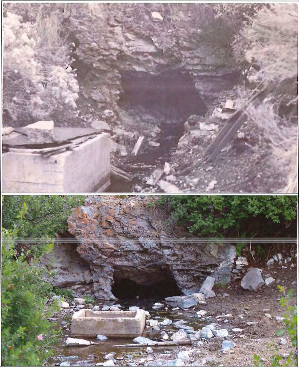
(Top) October 1962, discharge is estimated at less than 10 gpm. (Bottom) June 29, 2004, discharge is 0.022 cfs (10 gpm).
