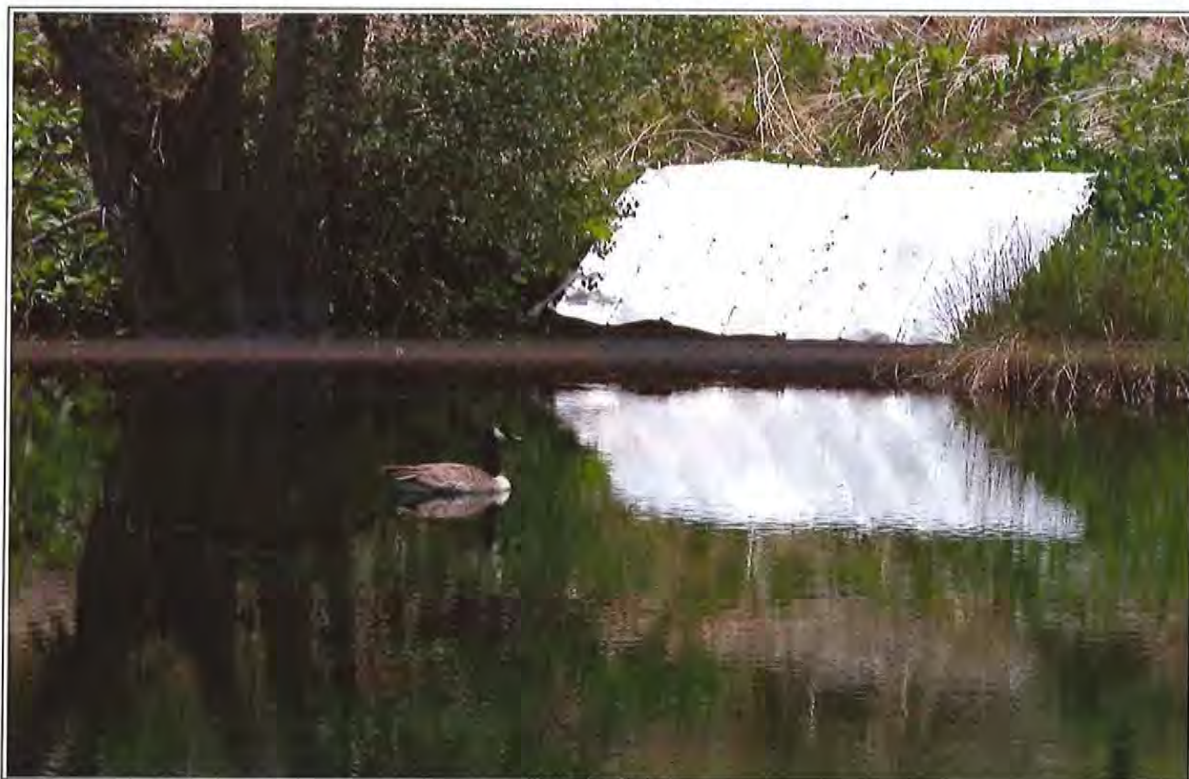
Figure 3-64 Hiko Spring Reservoir and Springhouse
