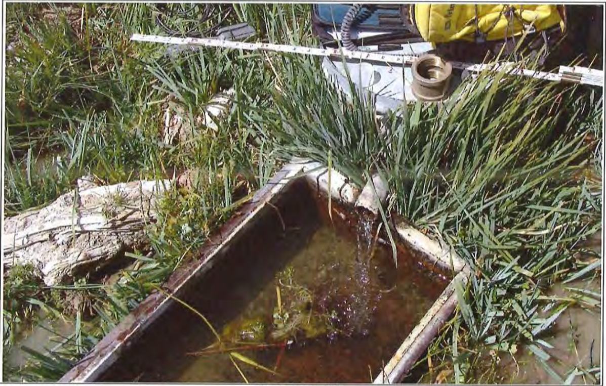
Figure 3-23 South Bastian Spring Diversion Appliances
