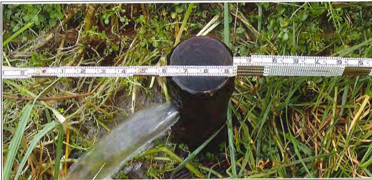
Figure 3-42 Discharge Pipe at Caine Spring
