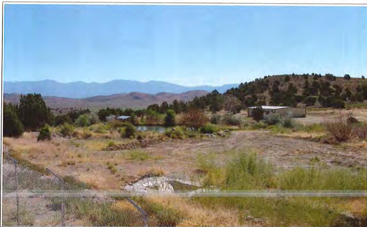
Spring orifice is in the concrete box in the foreground.
