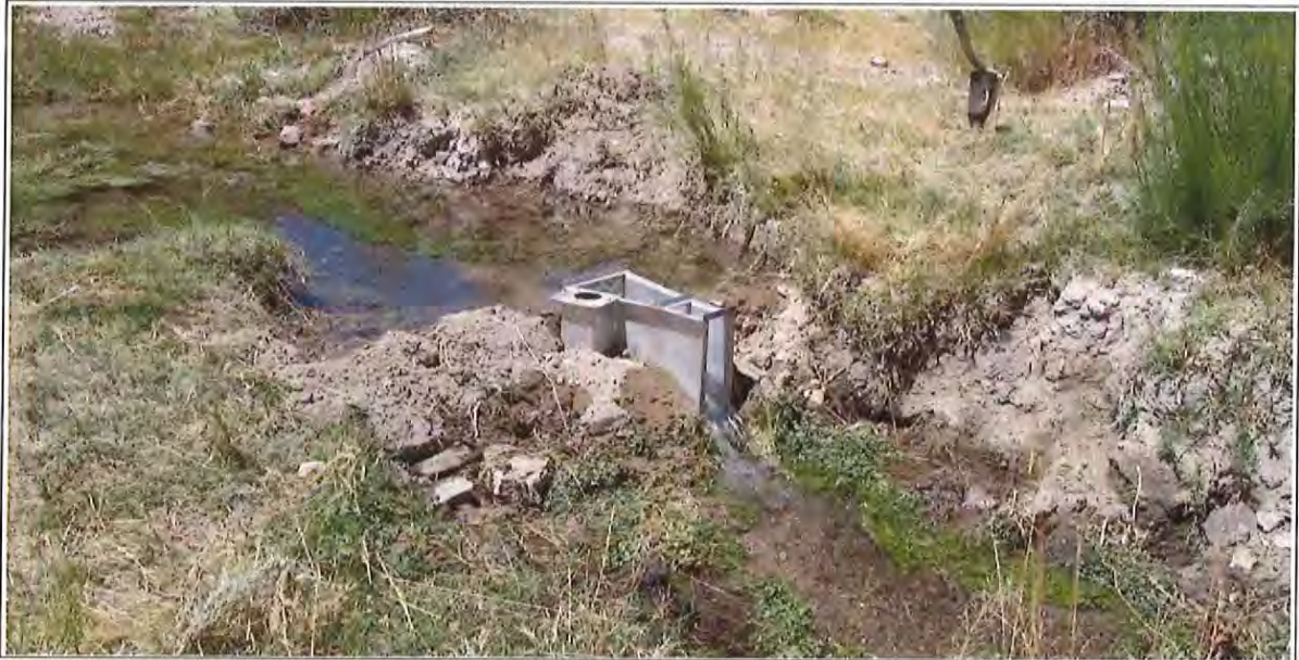
Figure 3-48 Three-Inch Modified Parshall Flume Installed 75 ft Downstream of Douglas Spring Orifice
