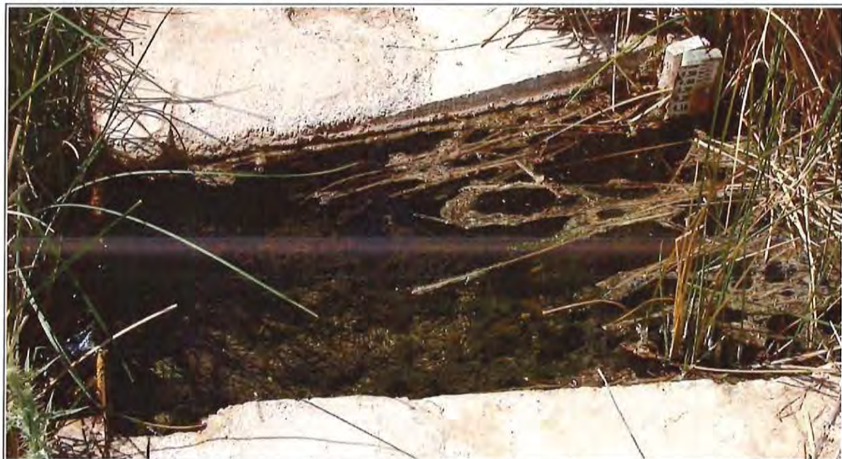
Figure 3-89 Blue Point Spring Weir Plate and Concrete Channel, Showing Heavy Algae Growth
