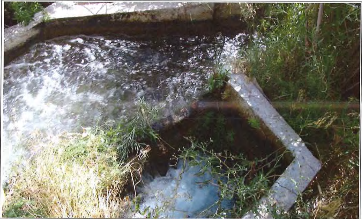
Figure 3-40 Second Splitter Box on Warm Springs Creek
