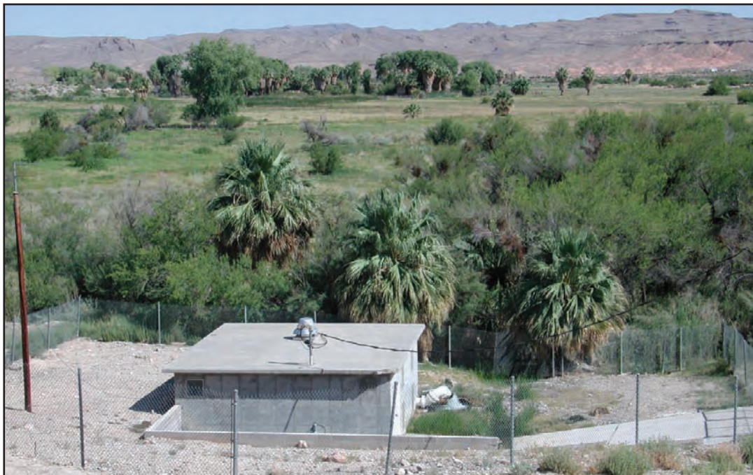
Figure A11. View of the Baldwin Springs area and the Moapa Valley Water District pump house in the Warm Springs area near Moapa, Nevada. Photographed in June 2004 by D. Beck.
