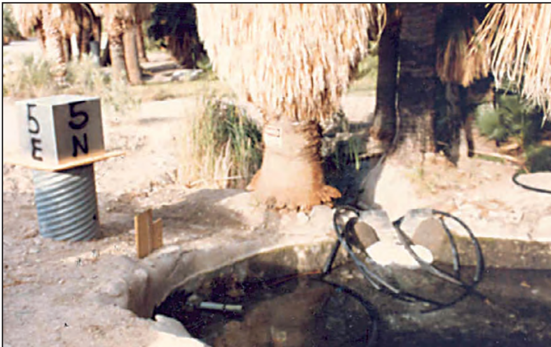
A. View of first weir being installed in 1986.
