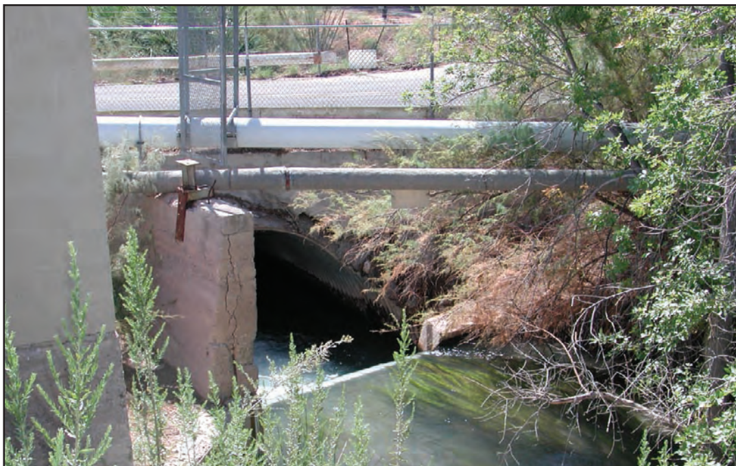
Figure B2. View looking downstream of the Cipolletti weir upstream of Warm Springs Road at the Muddy River stream-gaging station (09416000) in the Warm Springs area near Moapa, Nevada. Photographed in June 2004 by D. Beck.
