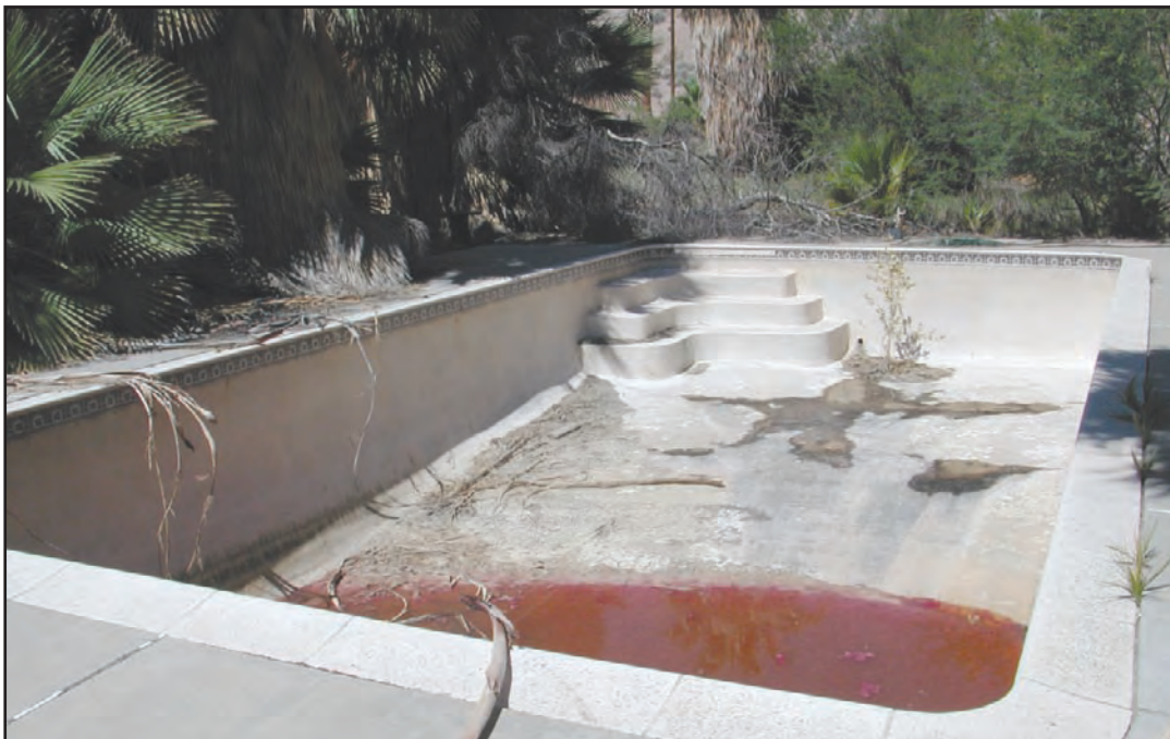
B. View of former swimming pool built by Frederick Apcar around 1980.
