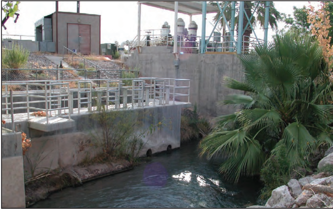
Figure A10. View looking downstream at Nevada Power Company water diversion and pumping station on the Muddy River, in the Warm Springs area near Moapa, Nevada. The diversion is about 100 feet upstream of the U.S. Geological Survey streamflow-gaging station at Warm Springs Road. Photographed in February 2004 by D. Beck.
