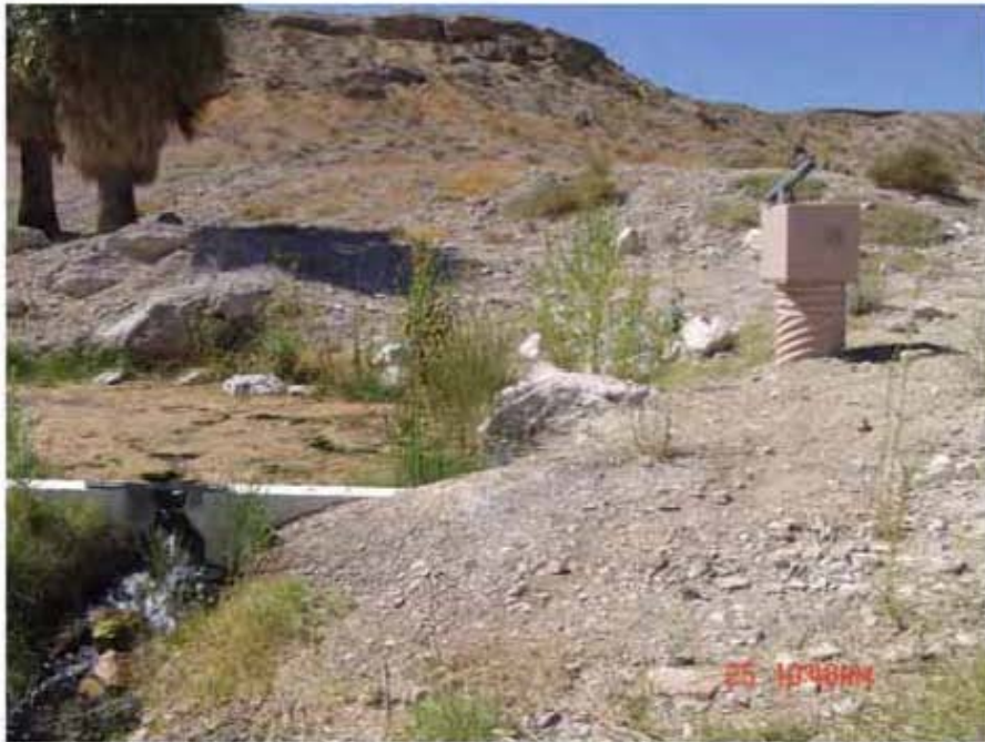
Figure 23 - Replacement Weir at Pederson Spring
