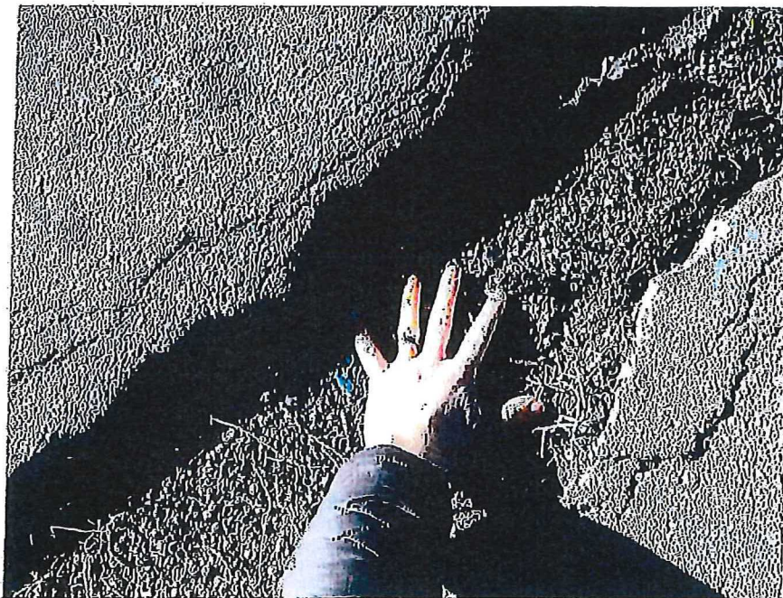
Figure 12 Magnitude of cracking on Newlands Drive February 1, 2014
