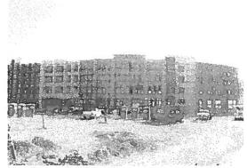
Building #2 west elevation - stucco lath and stucco scratch, brown and finish in progress
