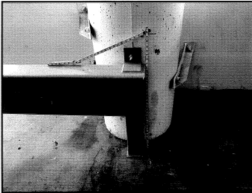
Photo 16: Repaired Spandrel Connections Configuration at Round Column (East End)
