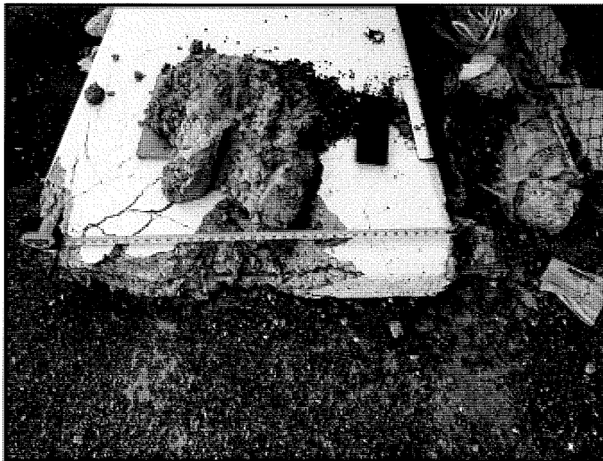
Photo 4: West End of Spandrel Barrier – Despoiled Anchor Failure Location
