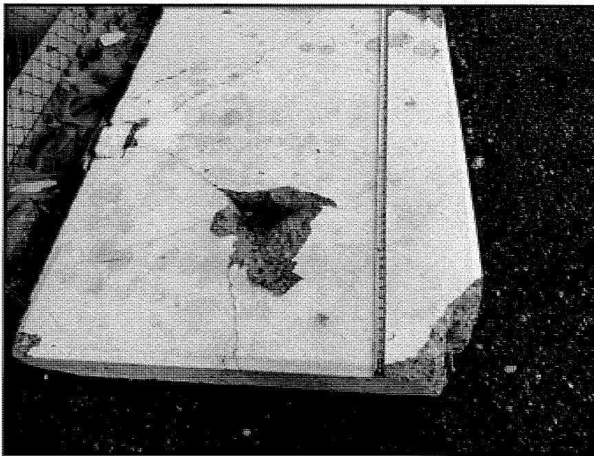
Photo 6: East End Retrofit Anchor Failure Location
