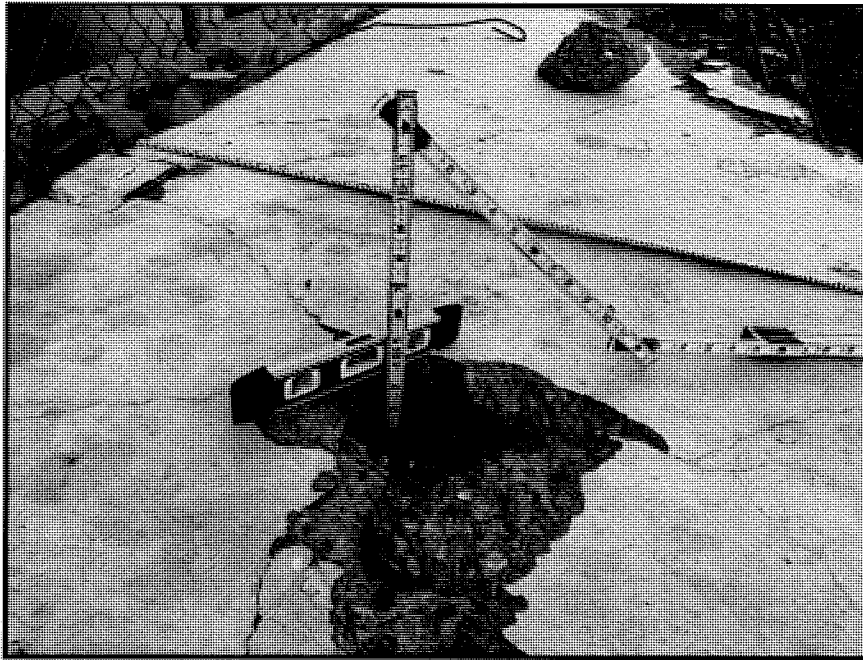
Photo 7: View of East End Spandrel Concrete Failure Depth at Retrofit Epoxy Anchor
