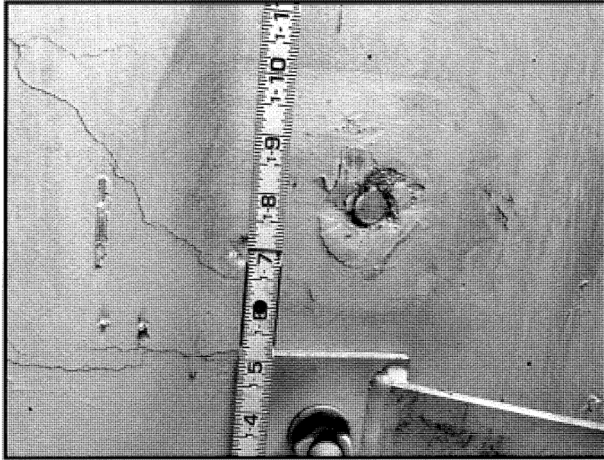
Photo 15: Cut-off Anchor in Rectangular Column at West End of Spandrel
