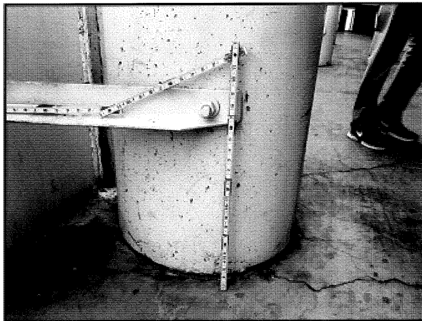
Photo 17: Repaired Lower Angle Panel Support at East End Round Column
