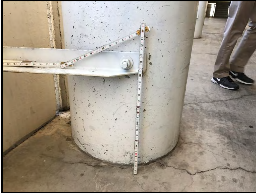
Photo 17: Repaired Lower Angle Panel Support at East End Round Column
