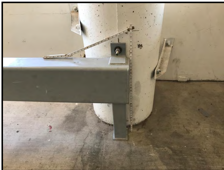
Photo 16: Repaired Spandrel Connections Configuration at Round Column (East End)
