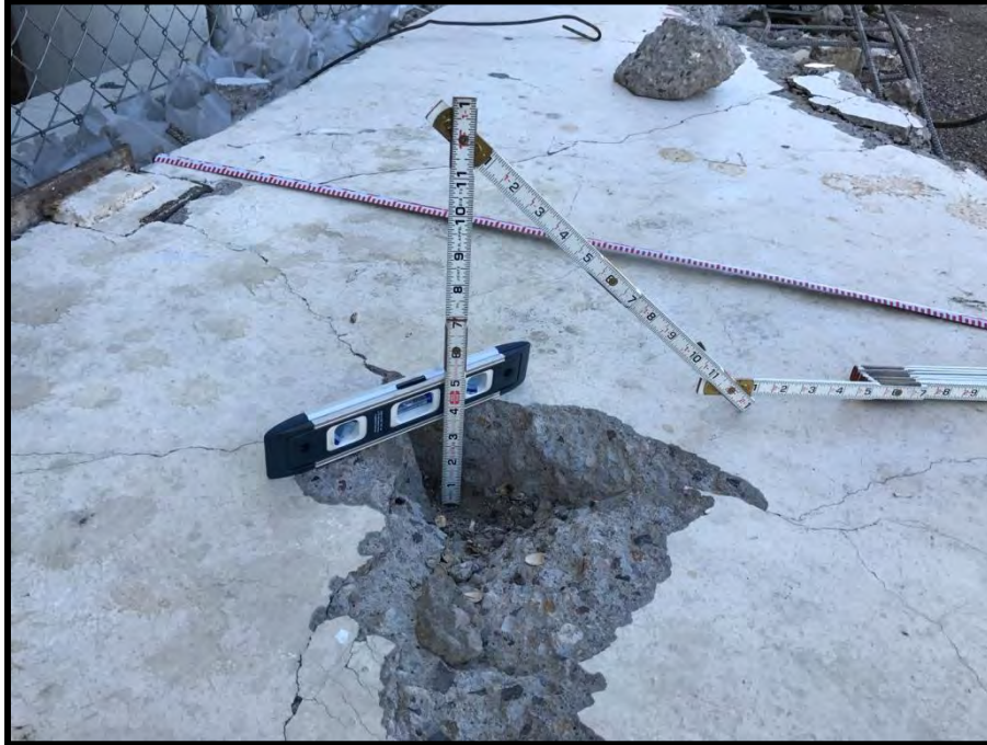
Photo 7: View of East End Spandrel Concrete Failure Depth at Retrofit Epoxy Anchor
