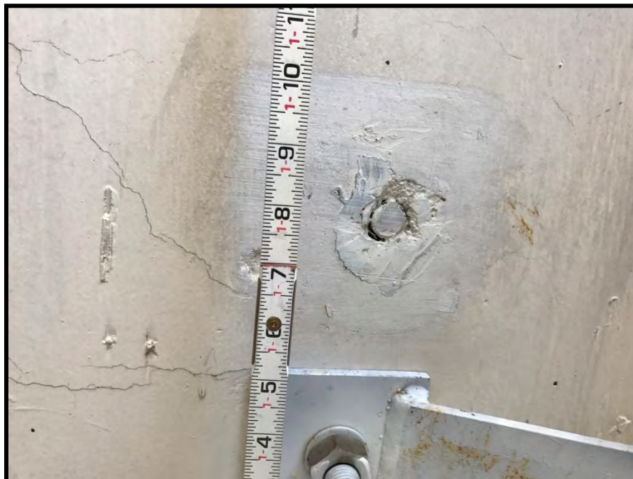
Photo 15: Cut-off Anchor in Rectangular Column at West End of Spandrel
