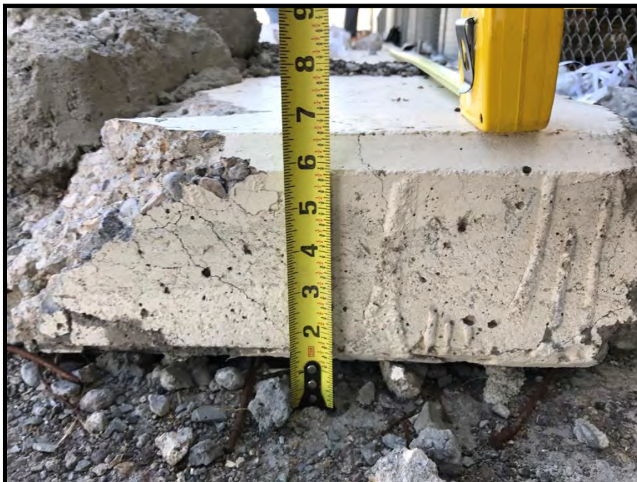
Photo 9: Measurement of Panel Thickness at West End of Spandrel
