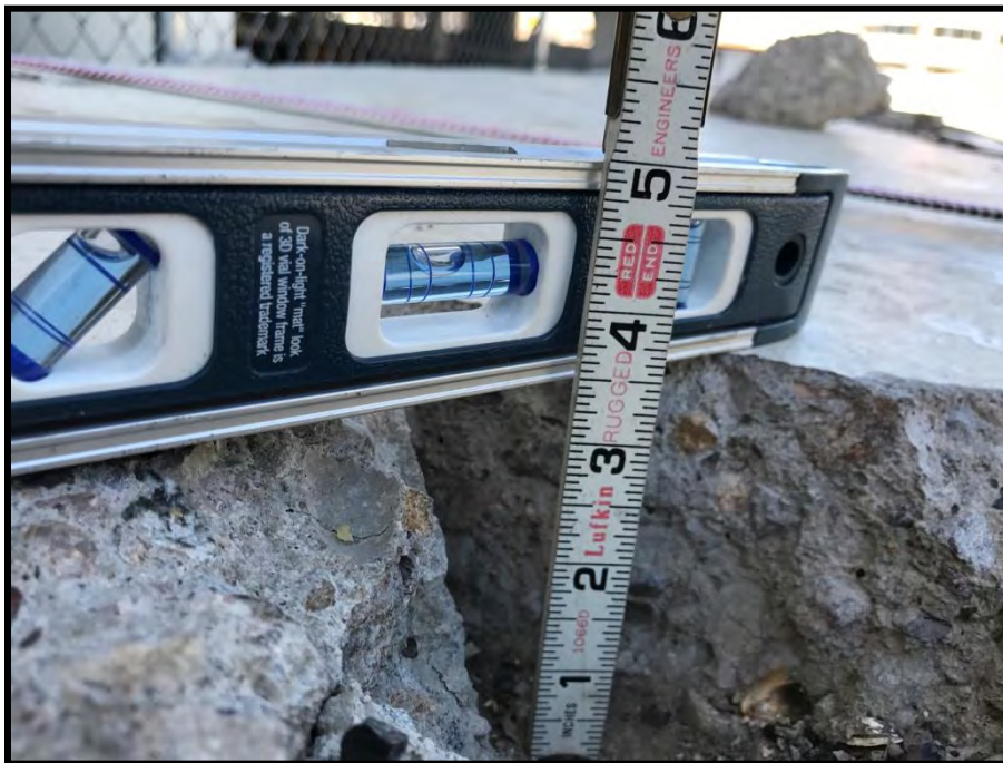
Photo 8: Approximate Depth Measurement of Concrete Failure
