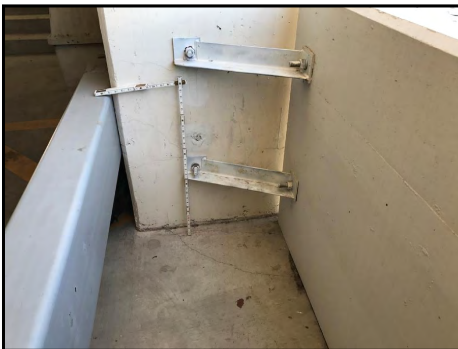
Photo 14: Repaired West End of Spandrel Barrier at Reif Crash Site
