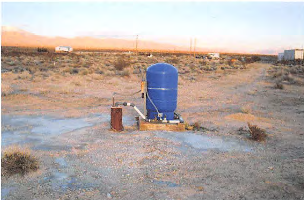
Photo 9. Typical domestic wellhead Photo credit: Tom Buqo, 2006
