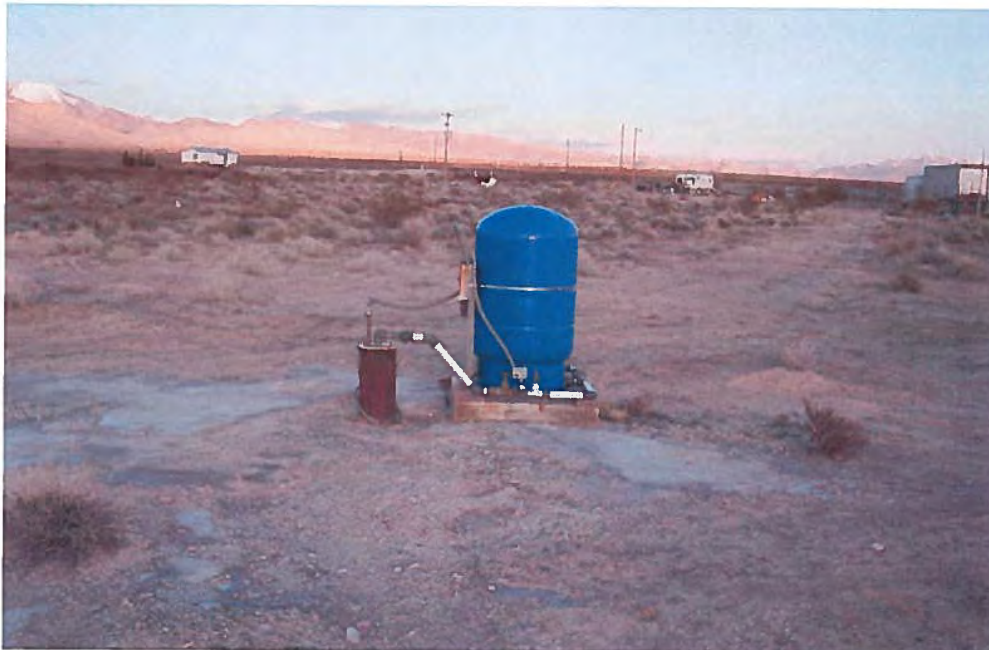
Photo 9. Typical domestic wellhead Photo credit: Tom Buqo, 2006
