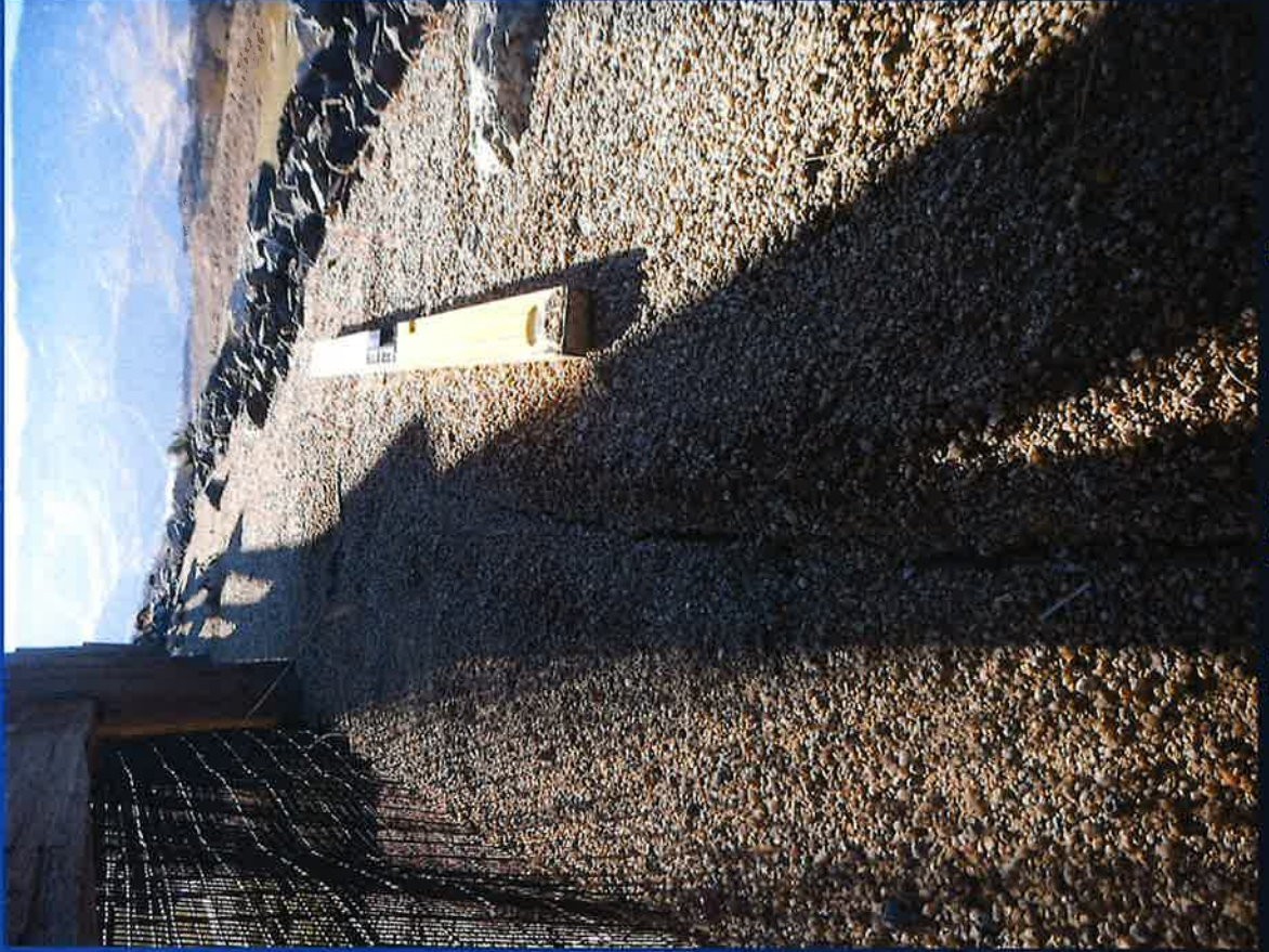
Soil crack behind rockery wall
