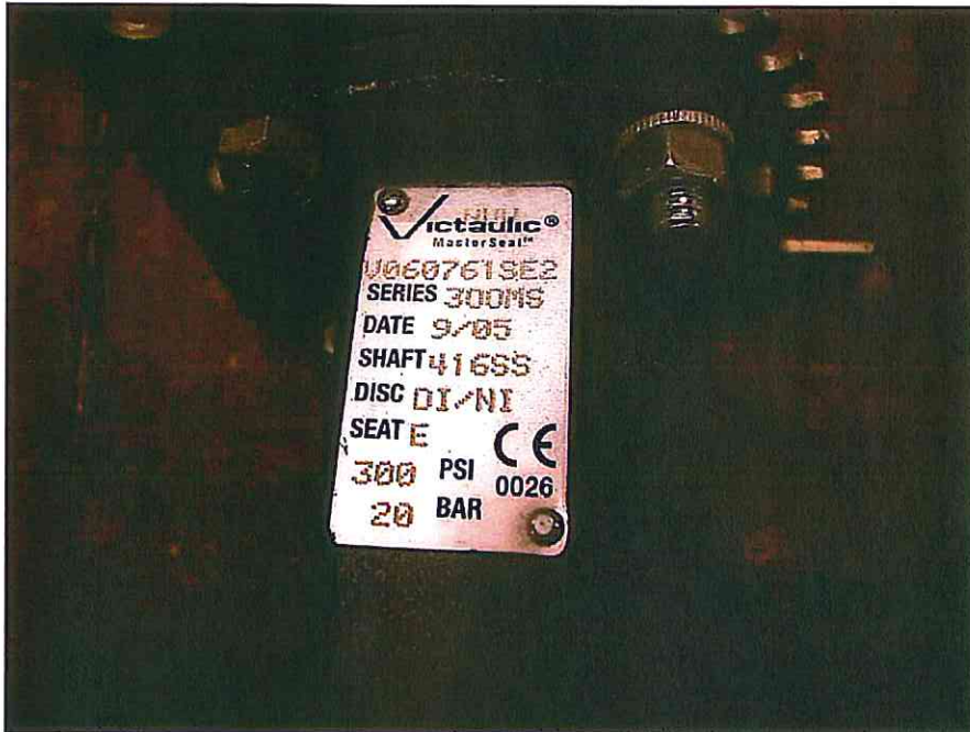
11. Name plate on typical carbon steel butterfly valve showing it has an AISI Type 416 stainless steel shaft; the ductile iron disc has a nickel edge (jpg34).
