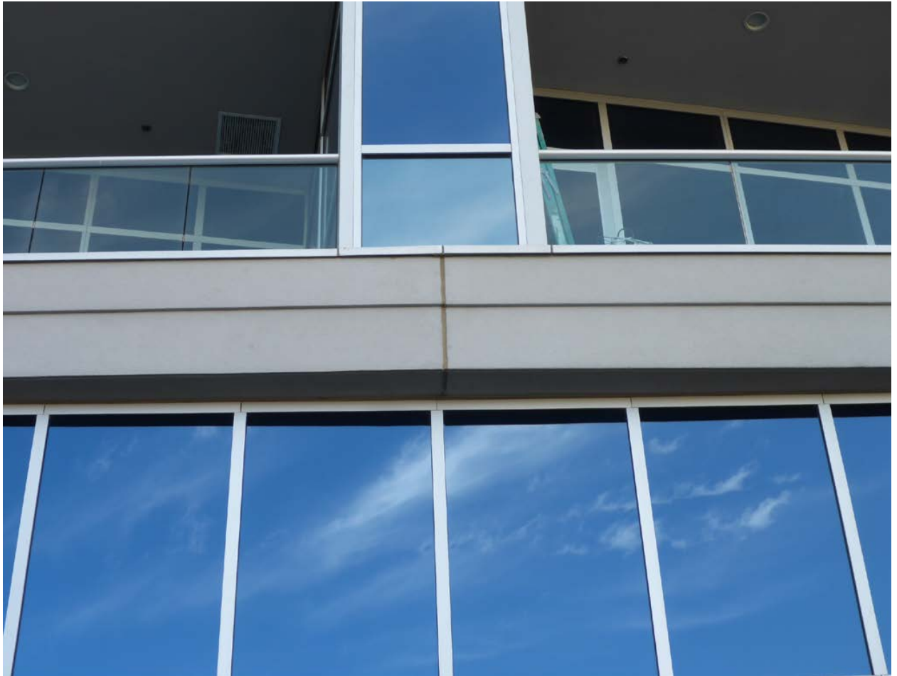
Exhibit 8 – ABBAE Photograph: View of the Tower Window System Showing Omission of Head Flashing
