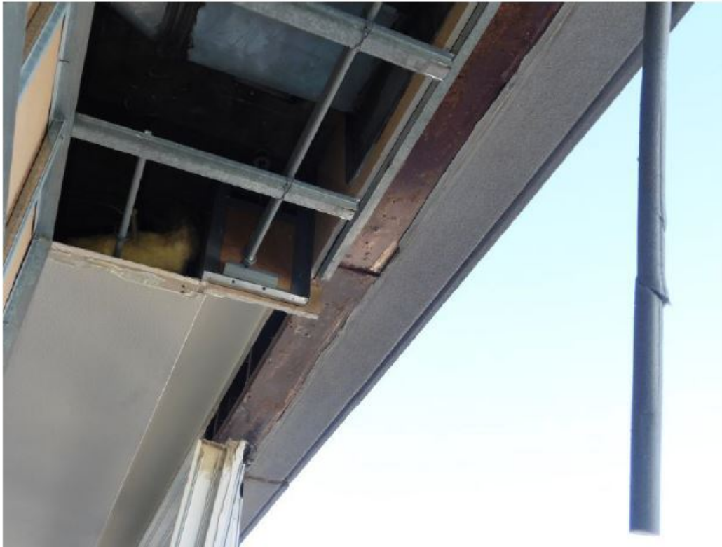
Exhibit 7 – CMA Consulting Photograph: Depicting Omission of Head Flashings
