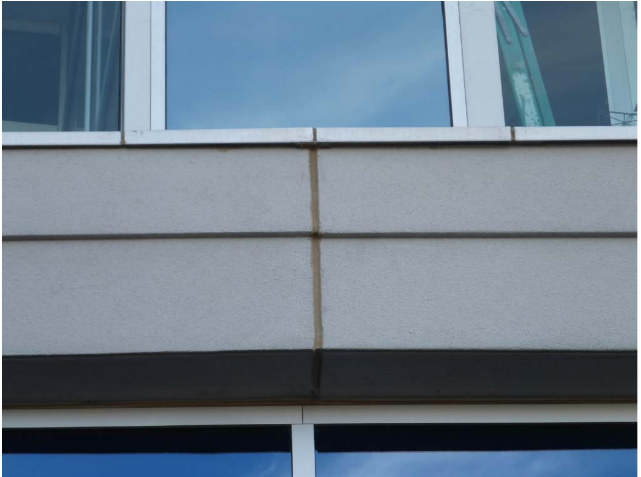
Exhibit 9 – ABBAE Photograph: View of the Tower Window System Showing Omission of Head Flashing
