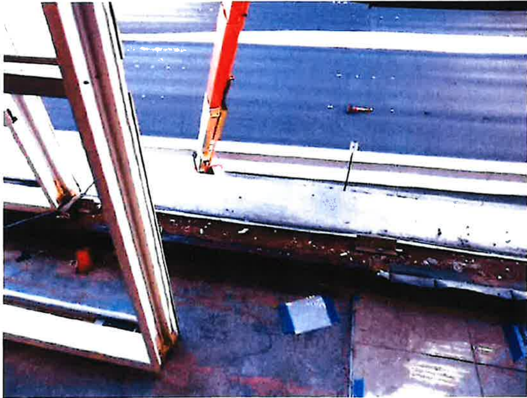
Exhibit 5 – CMA Consulting Photograph: Depicting Omission of Sill Pan Flashing
