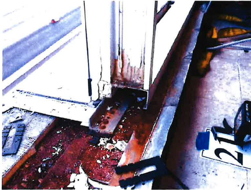
Exhibit 6 – CMA Consulting Photograph: Depicting Omission of Sill Pan Flashing
