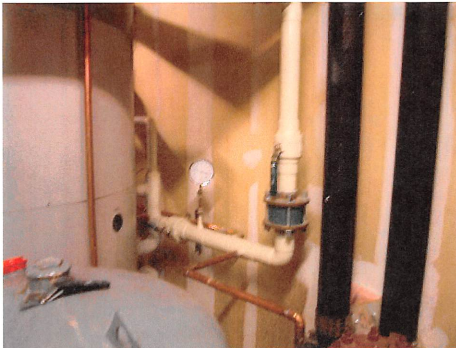
1. Hot water ferrous recirculation pump body requires replacement with a non-ferrous alloy now; replace carbon steel nipples now (jpg103).
