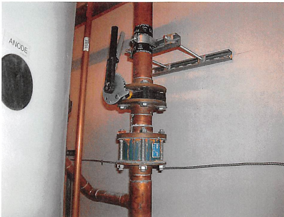
associated with Zone 1 hot water tank with steel butterfly valve and steel check valve (jpg47).
