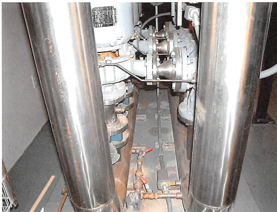
2. End view BP-1 skid mounted unit; stainless butterfly valves shipped with unit have been replaced with carbon steel valves that should be replaced now with stainless (jpg25).
