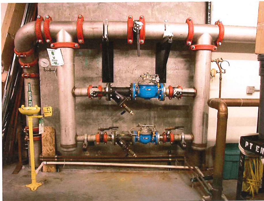
19. Lower pressure regulators; the far regulator is ductile iron top and bottom; the closer has a stainless steel top; visible residues at Unistrut are from connection leaks, not corrosion (jpg56).
