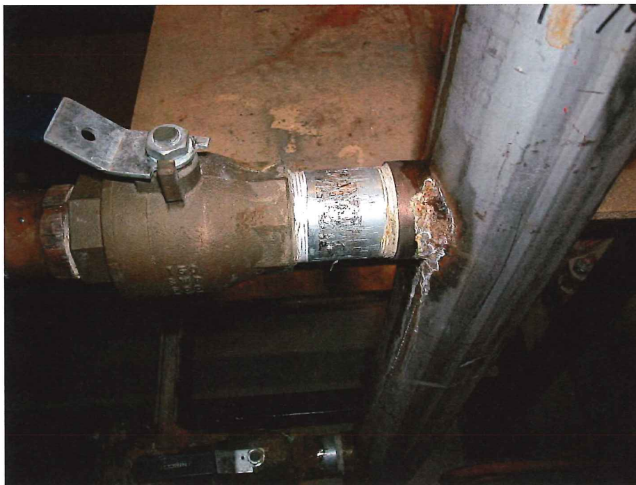
15. Carbon steel plastic lined nipple (lower southeast corner of manifold0 – replace with stainless steel (jpg52). Note: corrosion around Unistrut is a leak at the joint.
