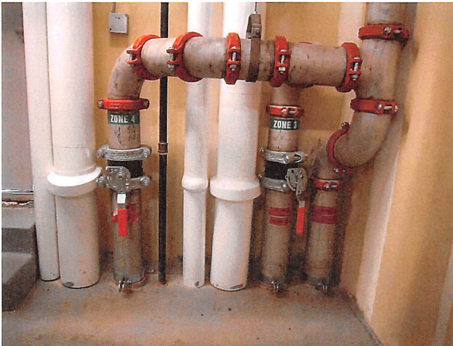
3. Zone 3 hot water system with 2 ferrous check valves that need to be replaced within 5 years.
