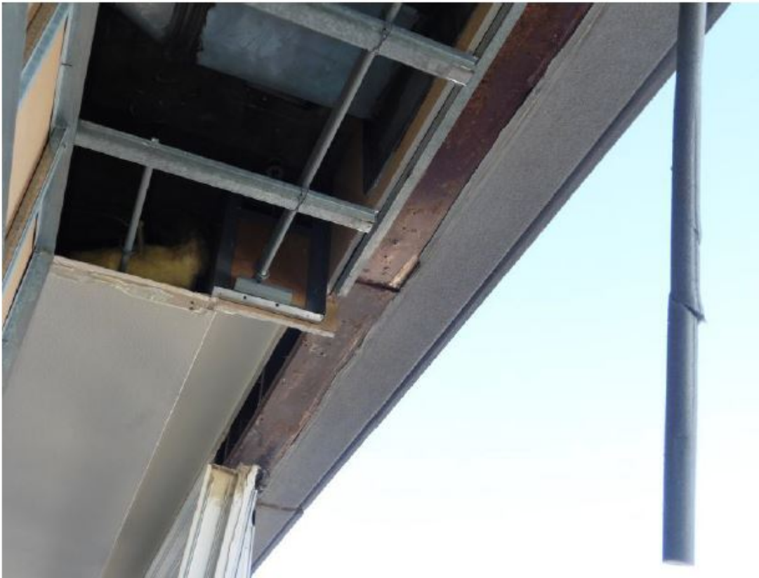
Exhibit 7 – CMA Consulting Photograph: Depicting Omission of Head Flashings
