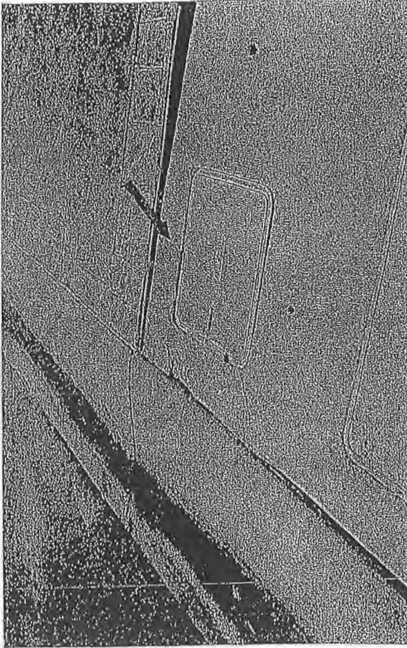
CRACKED AND CHIPPED CONCRETE UTILITY VAULT APRONS DEFECT 8
