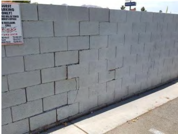
7. Damaged CMU perimeter wall
