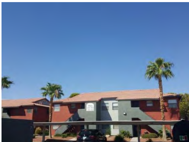
11. Stucco clad frontal façade with a Spanish tile gable and hip roof
