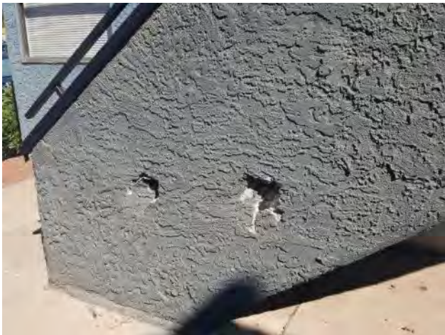
15. Punctured stucco covered stair system
