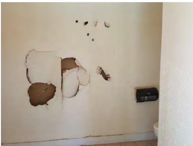
23. Damaged drywall in the pool toilet room
