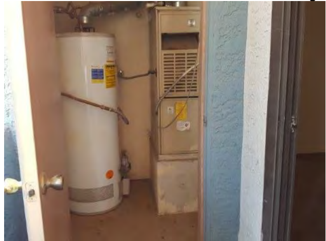
32. Hot water heater and furnace located in a utility closet accessed from the patio and balcony
