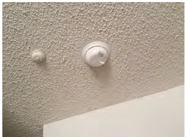
36. Smoke detector located in each apartment unit
