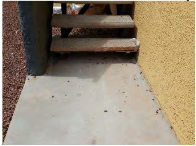
14. Broken concrete treads (repaired 10-9-2017)
