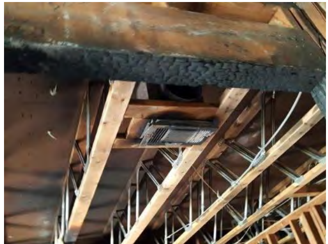
22. Open Web Joists in a fire damaged unit
