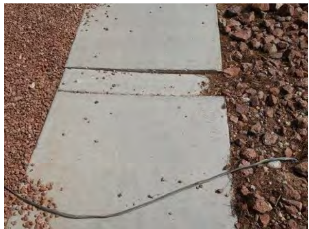
6. Uneven concrete sidewalk pavement (Repaired 10-17-2017)
