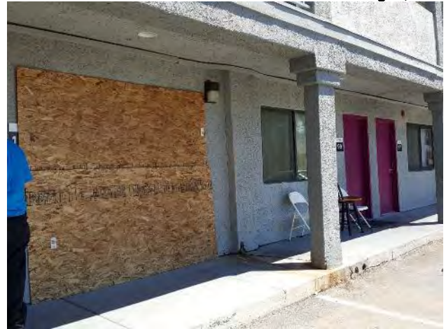
20. Unit 101's stucco clad sidewall exhibited excessive vehicular damage. Reportedly a car drove into the stucco clad sidewall. Plywood was observed over the window and sections of the wall.
