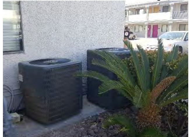
32. Several split system wall mounted air conditioning components were found to be old, not operating properly or not operational.
