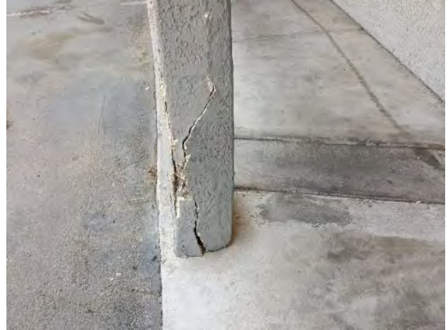
14. Stucco clad columns were found cracked and severely damaged. This condition was observed near Unit 9 and 377.
