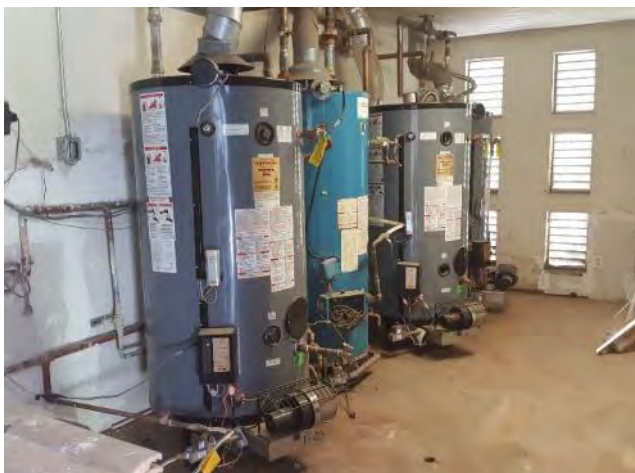
29. The Subject is provided with 6 natural gas-fired DHWHs.
