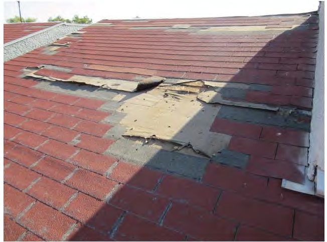
20. View of damaged composition asphalt shingled mansards.
