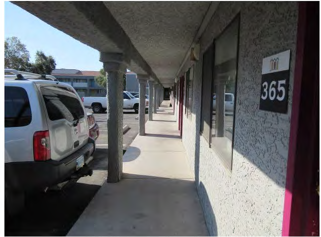
14. Building cladding includes painted stucco.
