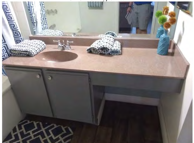
54. Bathroom vanities are wood with cultured marble counters and integral sinks.
