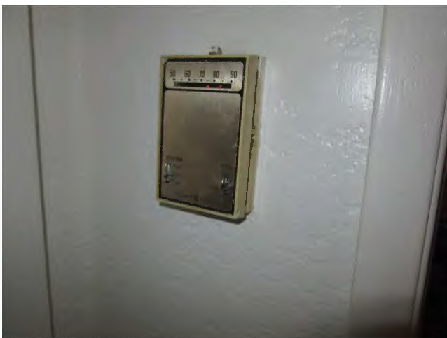
41. Wall-mounted manual thermostats control the temperature in each dwelling unit.
