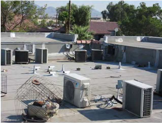
19. View of older modified bitumen roofing.
