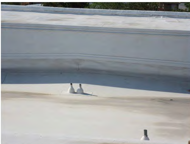
17. View of TPO roofing and flashing.
