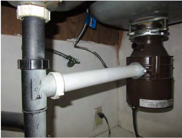
37. Drain lines are PVC.
