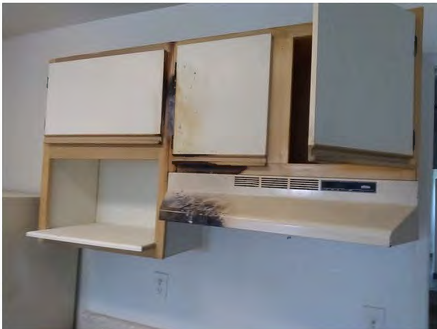
61. View of smoke/fire damaged kitchen cabinet and vent hood.
