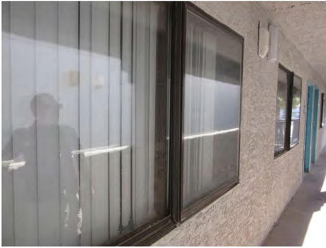
25. Building windows are double-pane sliding units in metal frames.
