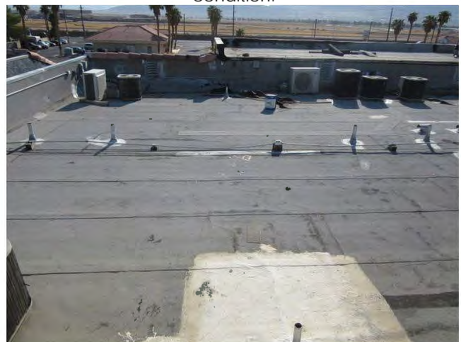
18. View of typical modified bitumen roofing on the east side buildings.
