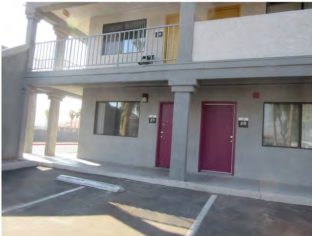
15. Building cladding includes painted stucco.
