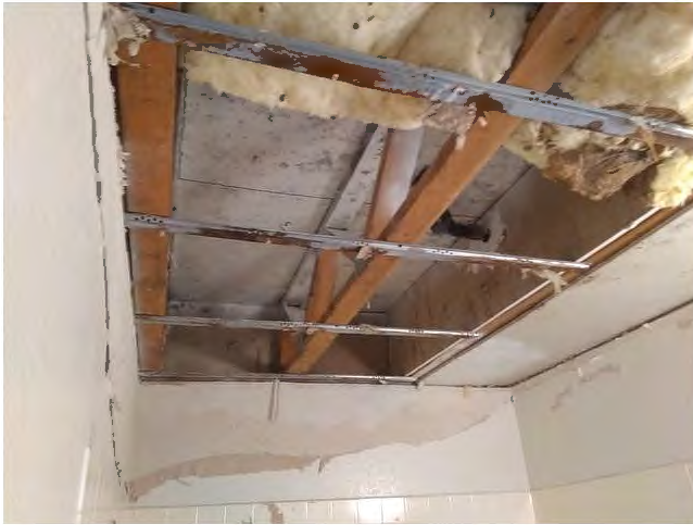
13. The buildings are conventionally wood framed (ceiling damage in a down unit is shown).
