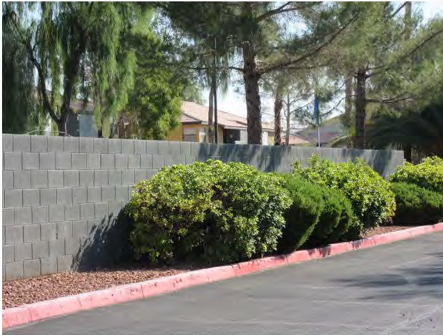
9. CMU fencing is present around the full perimeter of the Property.
