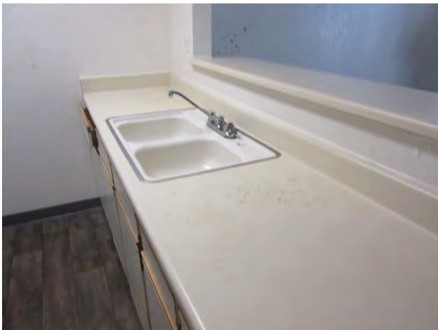
53. Kitchens counters are laminated plastic with porcelain or stainless steel sinks.
