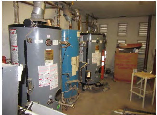
36. Central natural gas-fired water heaters also provide domestic hot water to the Property.
