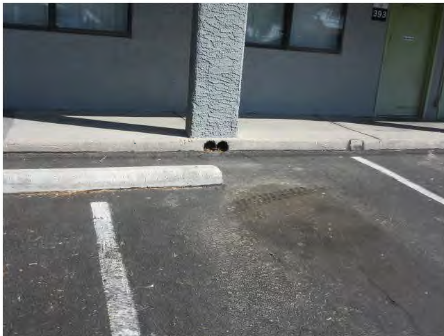
3. View of stormwater drain from an internal roof drain to the adjacent paved areas Storm water drainage is via sheet flow.
