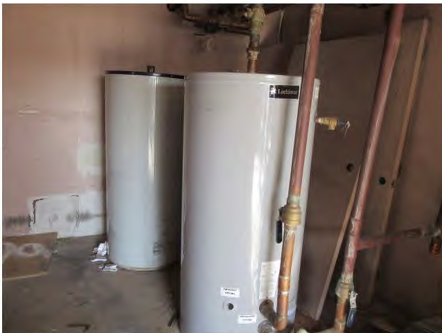
35. View of water storage tanks associated with the domestic boilers.
