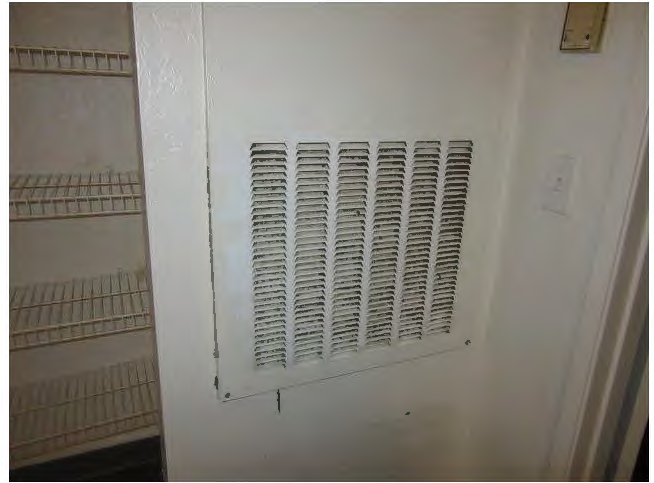
38. Air handlers with electric heating elements are mounted in the walls of the apartments.
