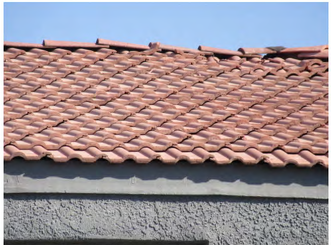
22. View of damaged concrete tiled mansards.
