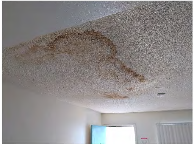
56. View of water-damaged ceiling in a vacant unit.
