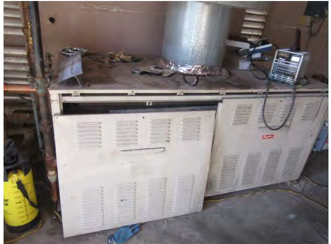
34. Heated domestic water is provided by domestic boilers and storage tanks. Building supply lines are copper.
