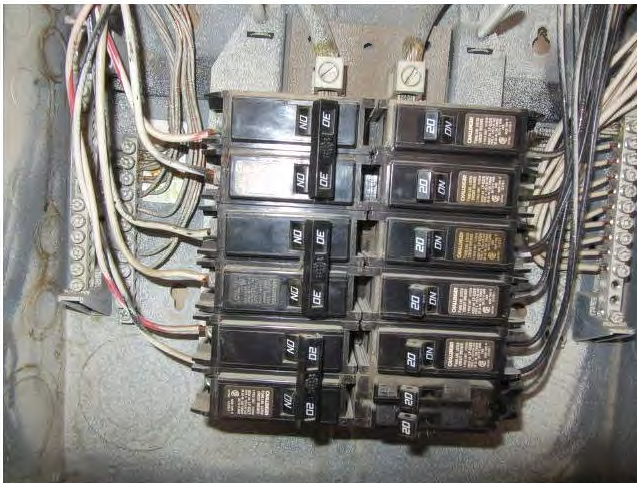
45. Branch wiring is copper.
