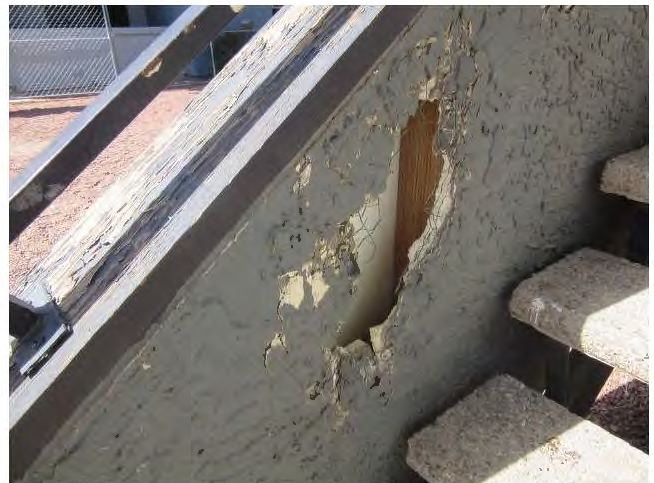
18. The stairway risers and handrails are damaged and paint is peeling at select locations.
