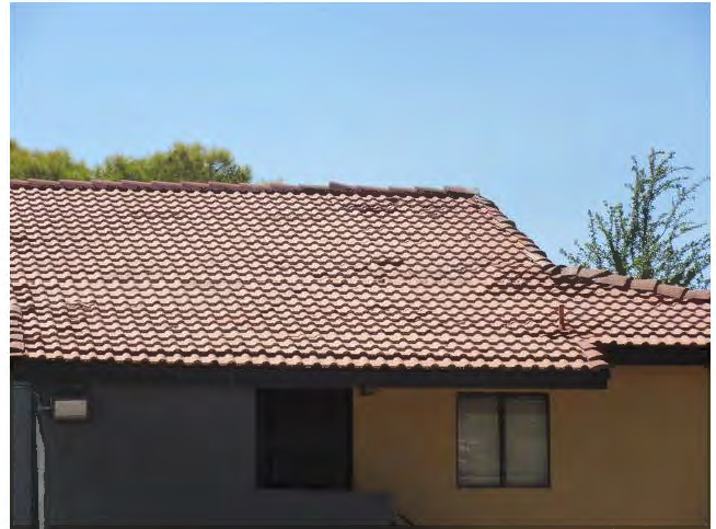
16. View of damaged concrete roof tiles.
