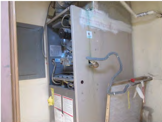
39. Heating in the units is provided via natural gas-fired furnaces.
