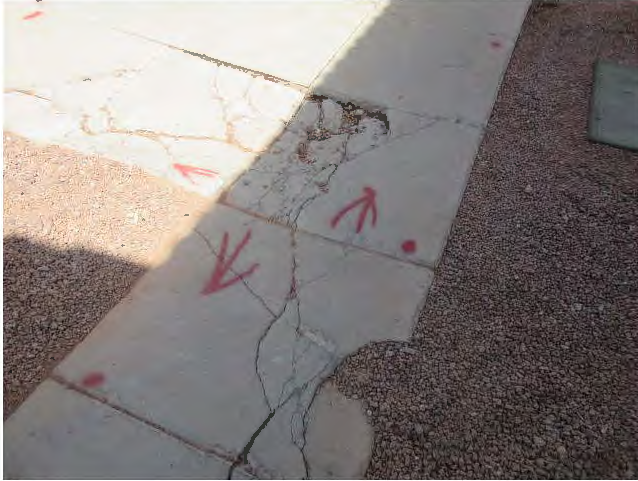
7. Concrete walkways provide access to the apartment buildings. Damaged and cracked areas of pavement were noted at select locations.
