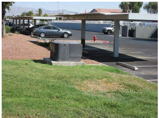
42. Power to the buildings is provided by pad-mounted transformers located throughout the Property.
