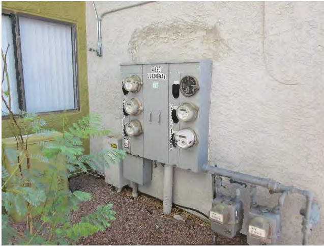
43. Electric service is individually metered.
