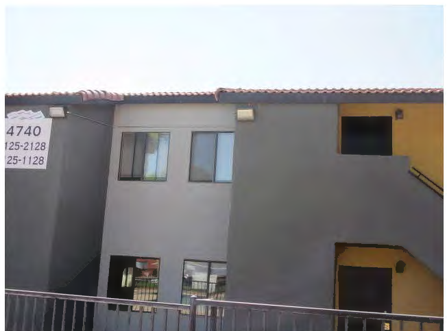
12. Building cladding includes painted stucco.
