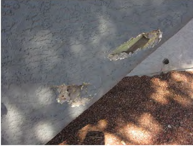
13. View of typical damaged stucco on the building exteriors.
