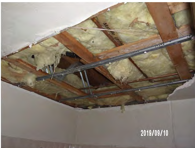
11. The buildings are conventionally wood-framed. Shown is a "down" unit.
