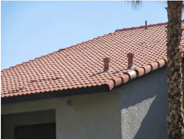
15. The pitched roofs of the apartment buildings are covered with concrete tiles (note damage).
