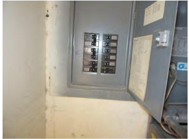
44. Breaker panels provide overload circuit protection.
