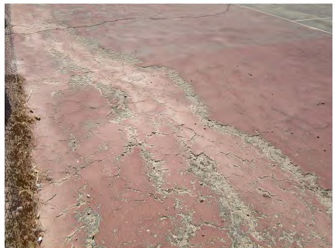
36. The sports court is cracked and damaged.
