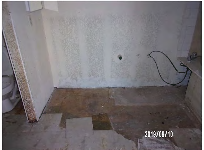
58. View of missing bathtub and damaged flooring in a down unit.
