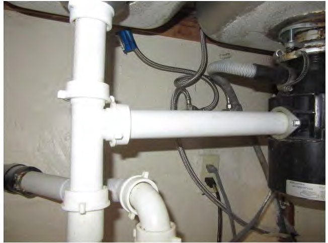
38. Drain lines are PVC.
