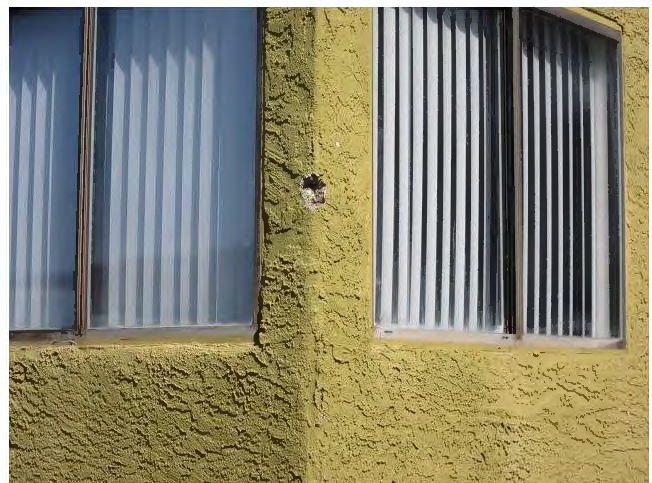
24. The building windows are double pane single-hung assemblies in metal frames.
