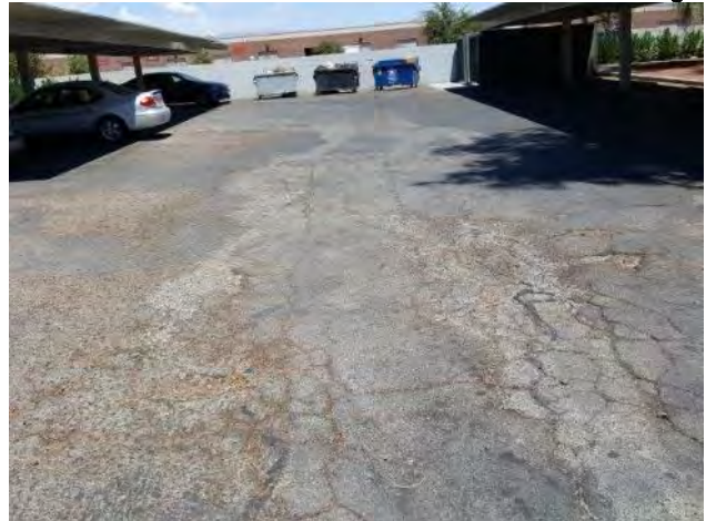
2. Severely damaged asphalt pavement
