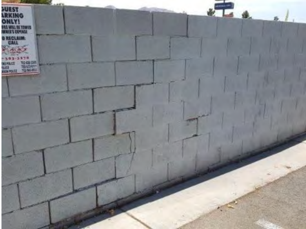
7. Damaged CMU perimeter wall
