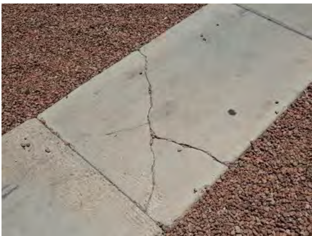
5. Cracks in concrete sidewalk pavement (Repaired 10-17-2017)
