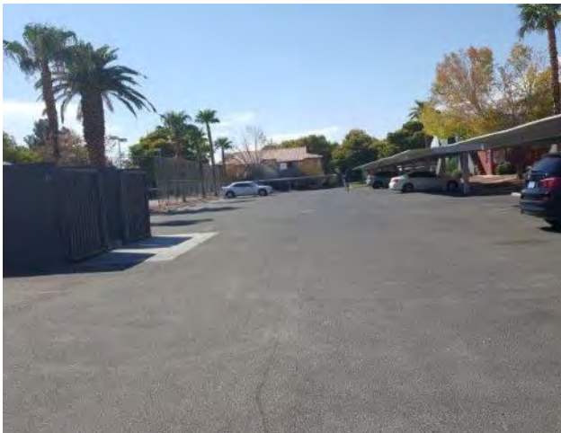
3. Asphalt pavement, steel framed carports and CMU refuse enclosure with steel metal gates
