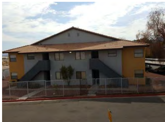
12. Stucco clad façade with a Spanish tile gable and hip roof and a metal tube fencing system.
