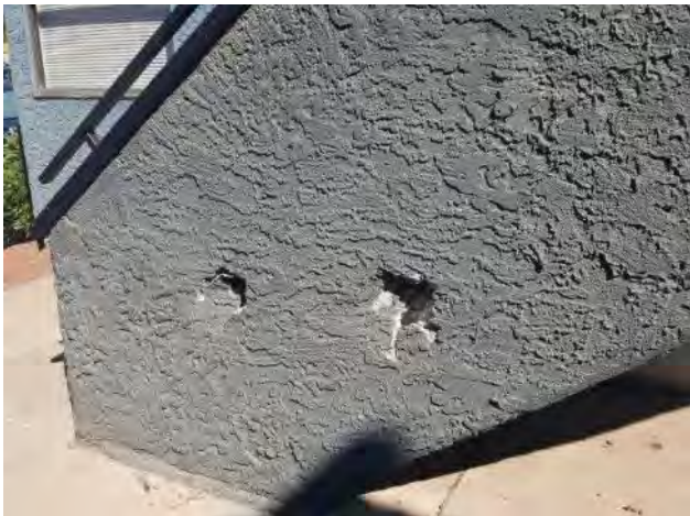
15. Punctured stucco covered stair system
