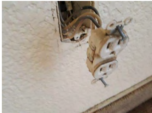
34. Open outlet verifying copper wiring
