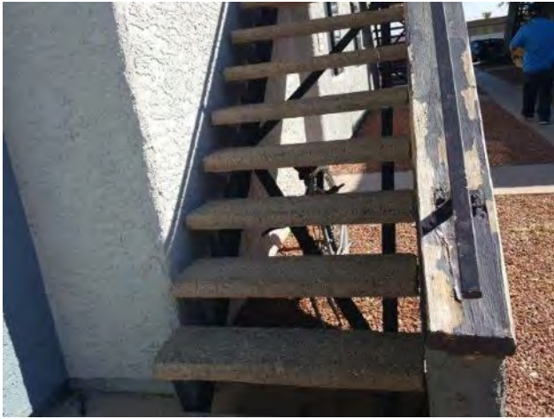
13. Dry rot on the wood handrail system
