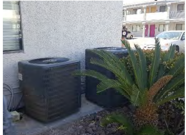
32. Several split system wall mounted air conditioning components were found to be old, not operating properly or not operational.
