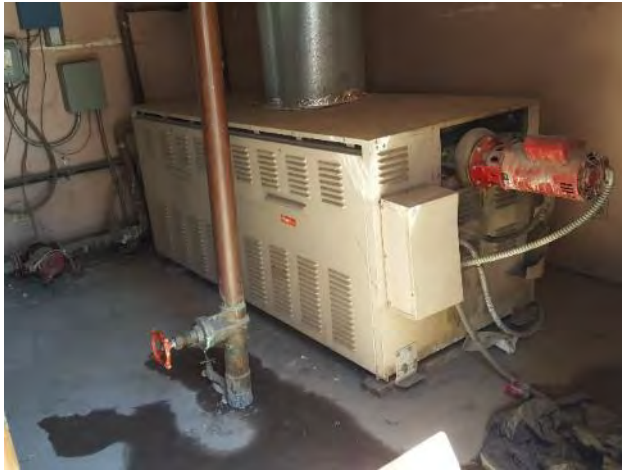
31. The Subject is provided with two natural gas-fired boilers manufactured by Raypak.
