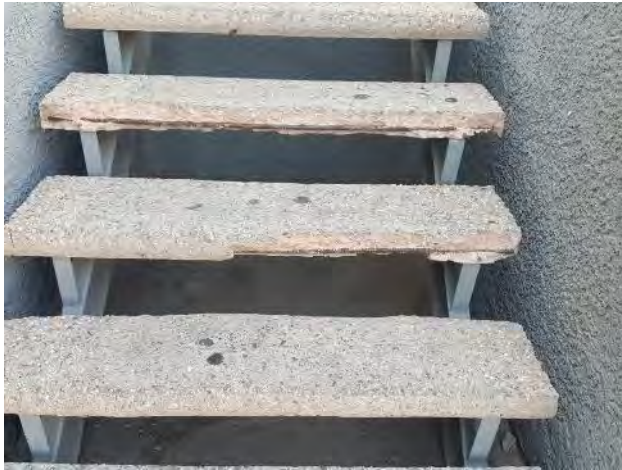
7. Stair systems exhibited excessive damage. Photographed above is an example of broken/missing metal corner boards. (Repaired 10-7-2017)
