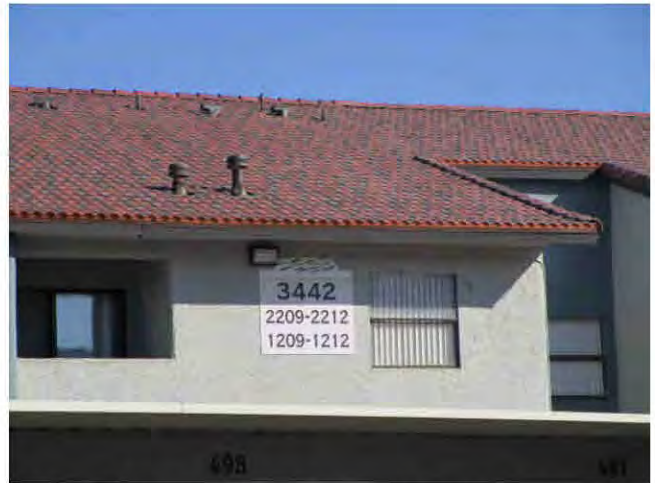
16. The pitched roofs of the apartment buildings are covered with concrete tiles.
