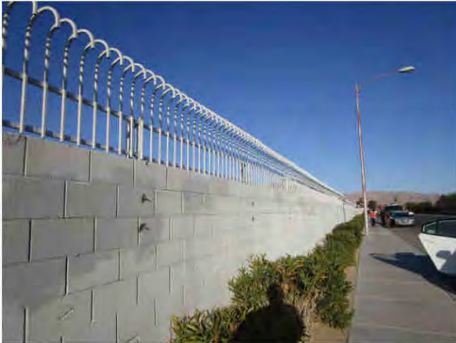
9. The Property is surrounded by a CMU wall. J-hooks have been added to the top for security purposes.
