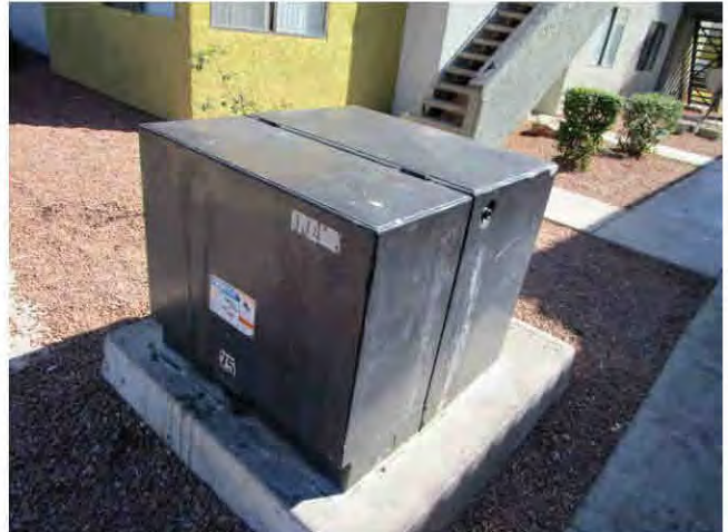
40. Power to the buildings is provided by pad-mounted transformers located throughout the Property.
