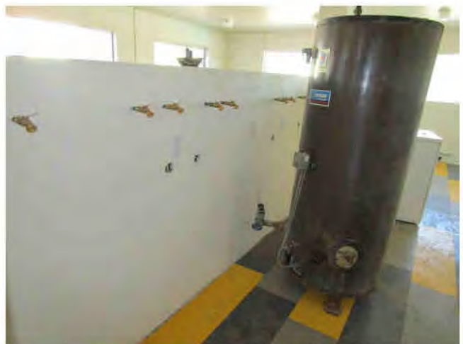
30. The water heater in the southwest laundry room has been disconnected.
