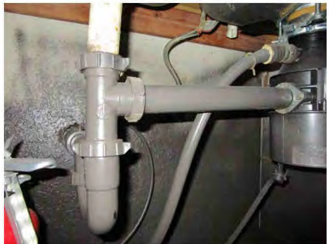
36. Drain lines are PVC.
