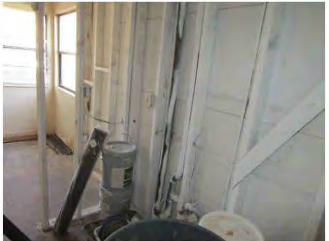
58. View of missing drywall in a down unit.
