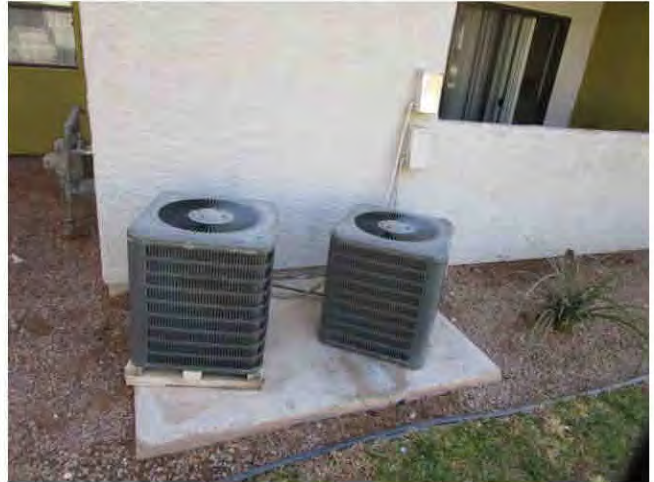
38. Cooling in the units is provided via pad-mounted A/C condensing units.
