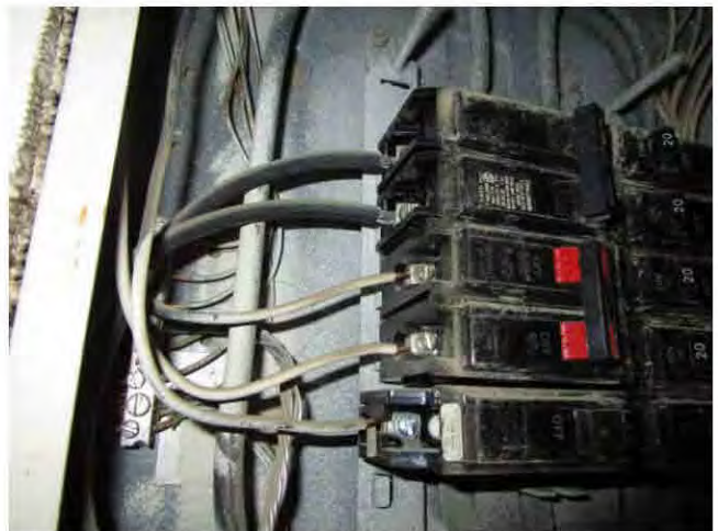
42. Breaker panels provide overload circuit protection.
