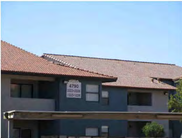
15. The pitched roofs of the apartment buildings are covered with concrete tiles.
