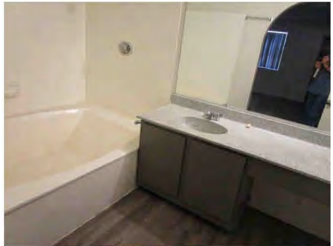
52. Bathtubs are fiberglass with ceramic tile shower surrounds.
