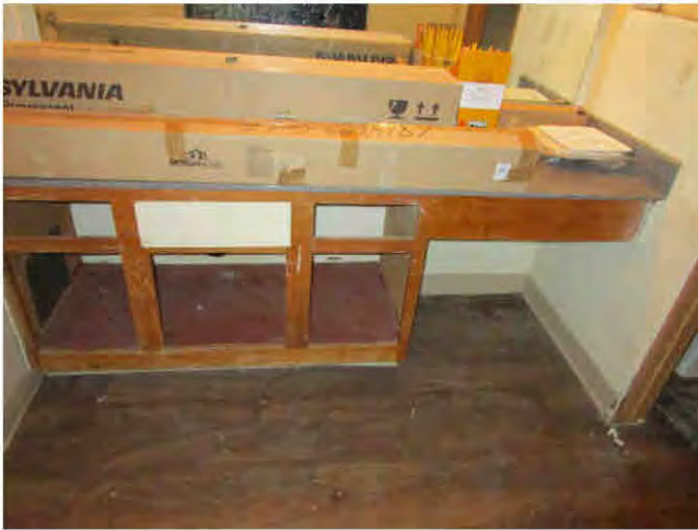
55. View of damaged vanity and partially removed drywall in a down unit.
