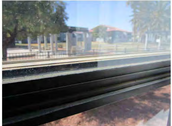
22. Building windows are double pane single-hung assemblies in metal frames.
