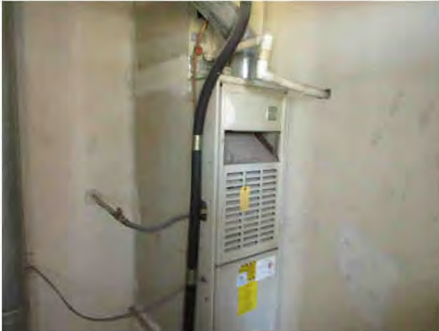
37. Heating in the units is provided via natural gas-fired furnaces.
