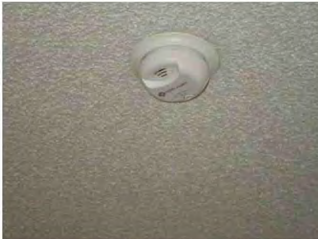
45. Smoke and CO detectors are installed in each dwelling unit.
