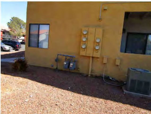
41. Electric service is individually metered.
