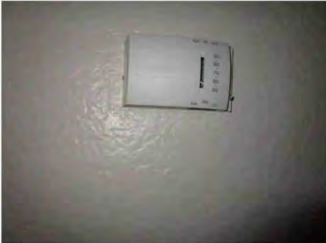
39. Temperature in the units is controlled by manual wall-mounted thermostats.
