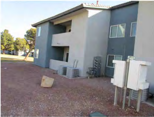
13. Building cladding includes painted stucco.
