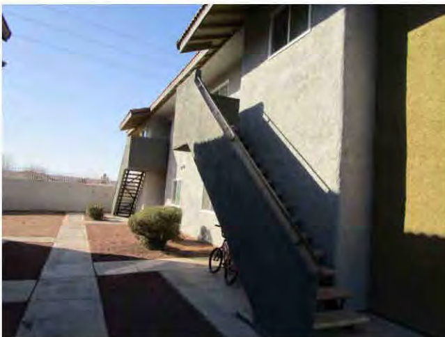
17. Steel-framed exterior stairs with stucco covered risers and railings provide access to the upper floor apartments.
