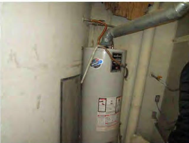
35. Domestic hot water is provided by individual natural gas-fired water heaters.
