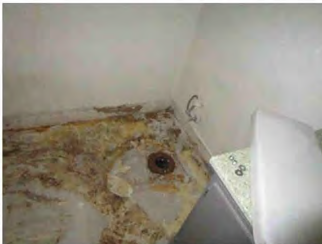
59. View of missing commode in a down unit.
