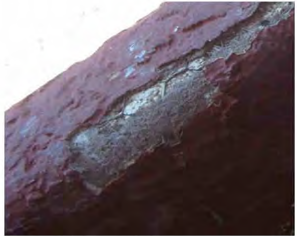
14. View of damaged stucco on a stairway handrail.
