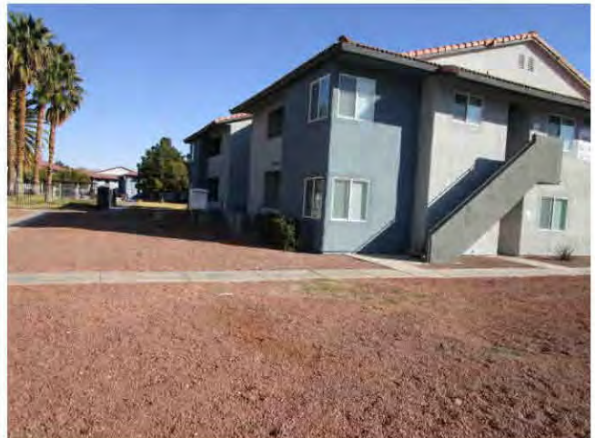
12. Building cladding includes painted stucco.
