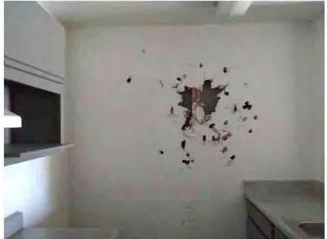
46. View of damaged wallboard in a vacant unit.
