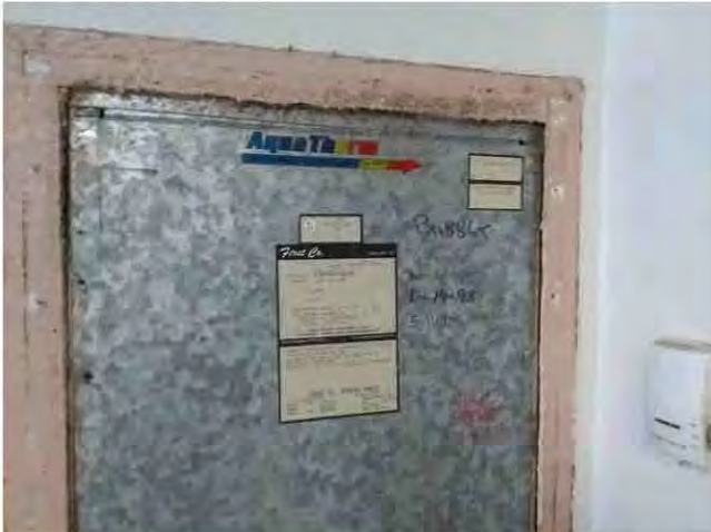
33. Heat in the units is provided by wall-mounted air handlers with electric heating elements.
