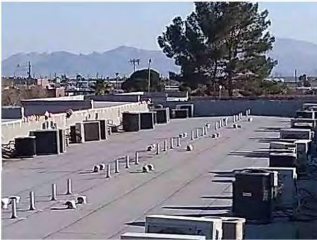
13. The flat roofs on the east side of the Property have modified bitumen roof coverings.
