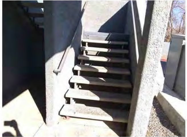
20. Upper floor units are accessed from exterior stairways with precast concrete treads.
