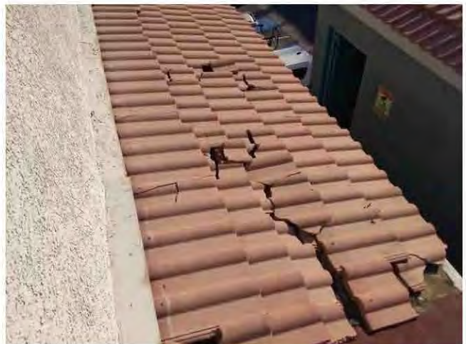
18. View of damaged concrete tiled mansards.
