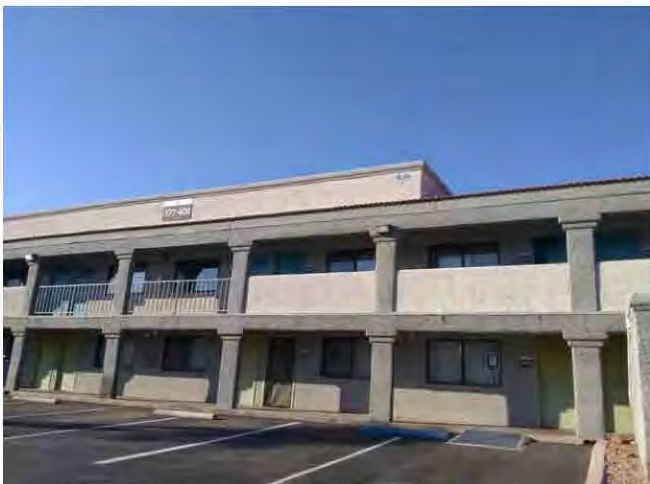
11. Building cladding includes painted stucco.
