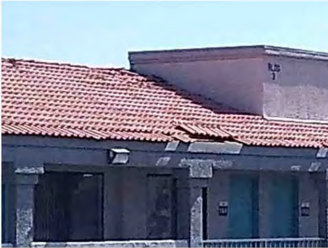
19. View of damaged concrete tiled mansards.
