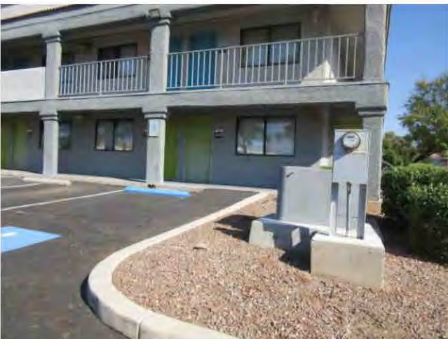
35. Pad-mounted electric transformers provide power to the buildings (note master meter).
