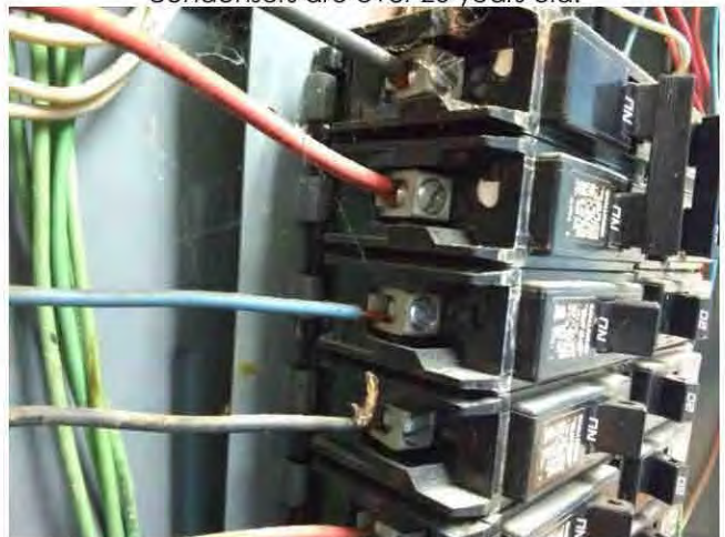
36. View of a building circuit breaker panel providing overload protection. The branch wiring is copper.
