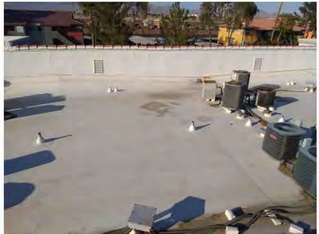
16. Typical TPO membrane roofing.
