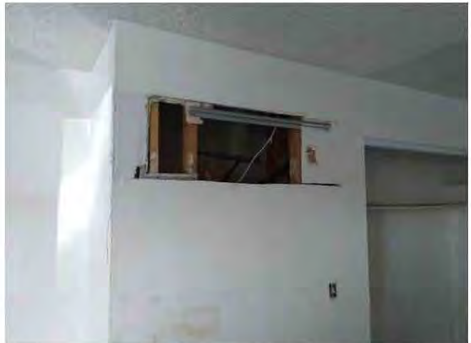
10. The two story buildings are wood framed (vacant unit shown).
