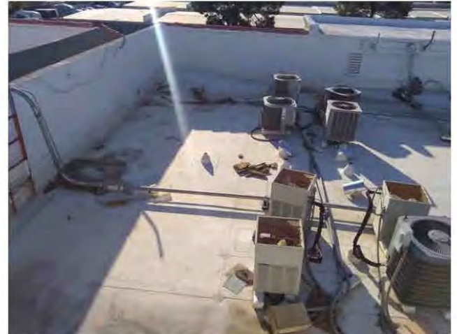
34. Cooling to the dwelling unit is provided by roof-mounted A/C condensers. Approximately half of the condensers are over 20 years old.
