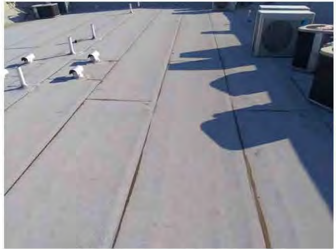
14. Typical modified bitumen roofing.
