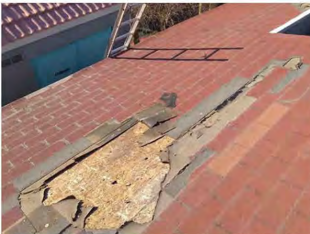
17. View of damaged composition asphalt shingled mansards.
