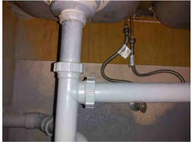
32. Building drain lines are PVC.
