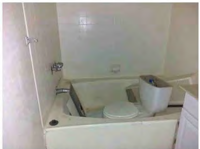
54. View of disconnected commode in down unit 105.
