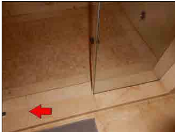
204. Tile loose, broken or missing tile
