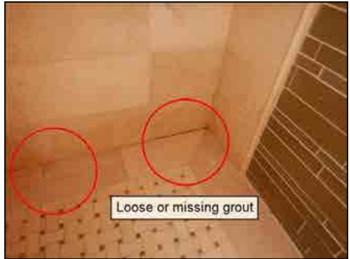
206. Tile loose, broken or missing tile
