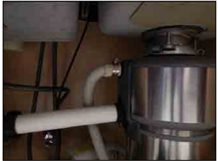
332. Backflow prevention missing
