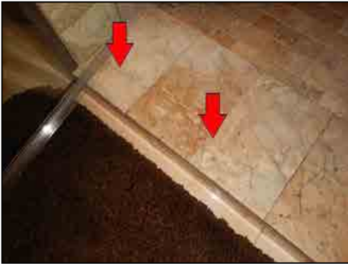
208. Tile loose, broken or missing tile
