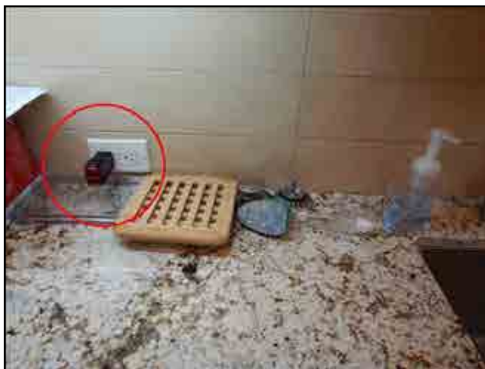
111. Test faulty on GFCI/GFI (Ground Fault...
