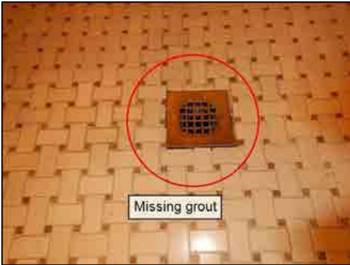
205. Tile loose, broken or missing tile
