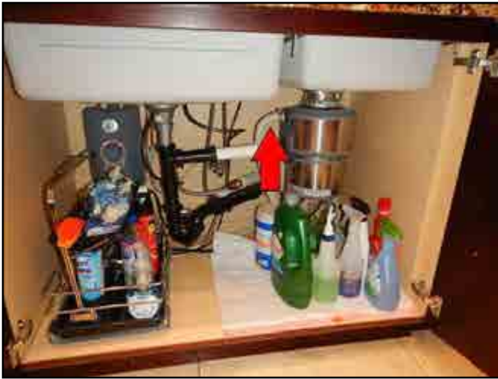
331. Backflow prevention missing
