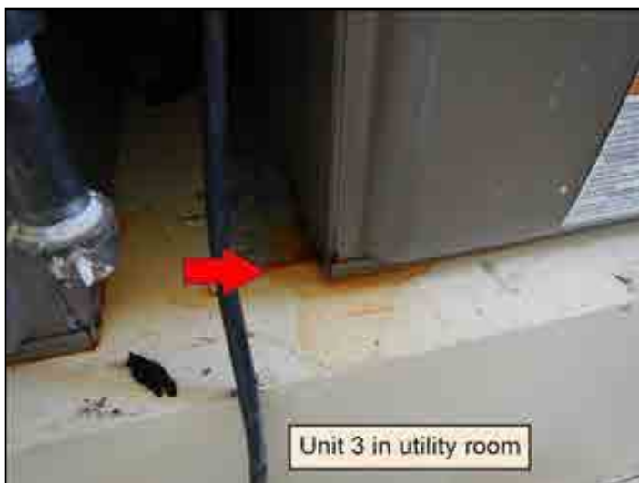
159. Condensate leak
