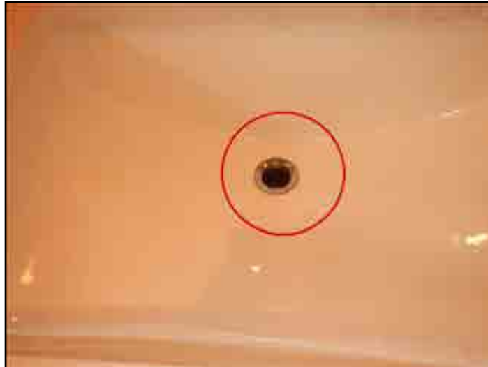
185. Drain stop missing
