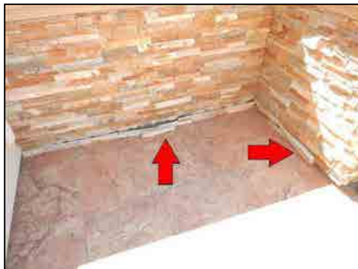
46. Masonry deterioration
