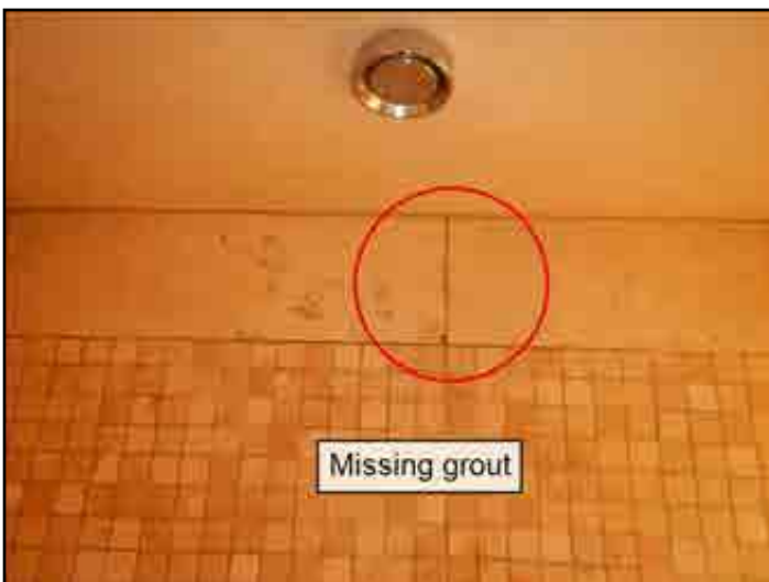
200. Tile loose, broken or missing tile
