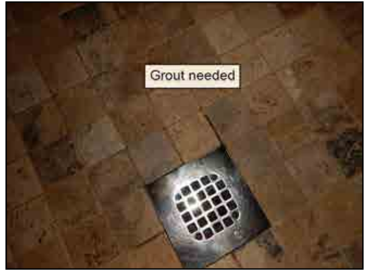
209. Tile loose, broken or missing tile
