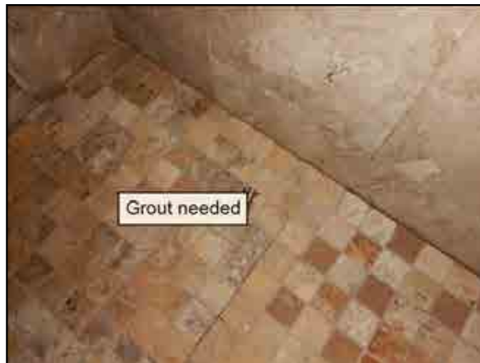
210. Tile loose, broken or missing tile
