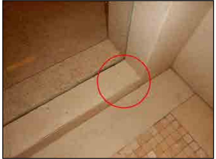
203. Tile loose, broken or missing tile
