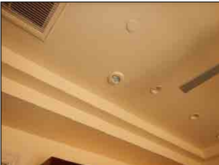
121. Missing smoke alarm
