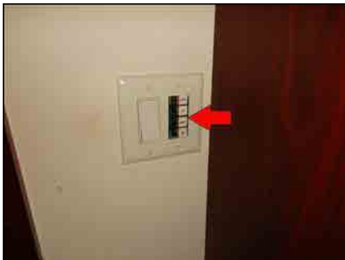
113. Damage cover plate
