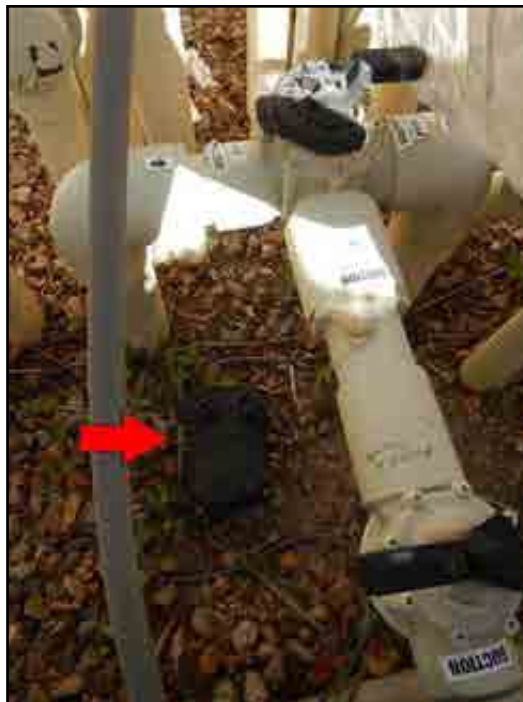
345. Automatic valve removed
