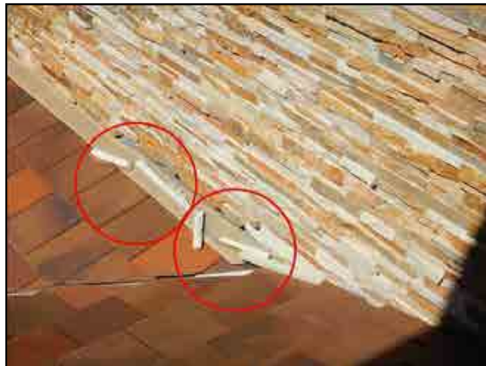
44. Masonry deterioration
