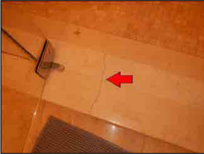
202. Tile loose, broken or missing tile
