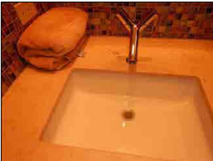
186. Drain stop missing
