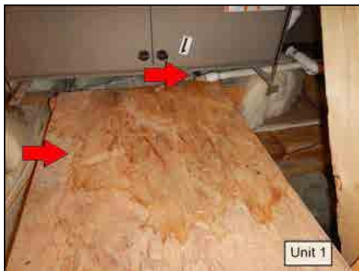
160. Condensate leak
