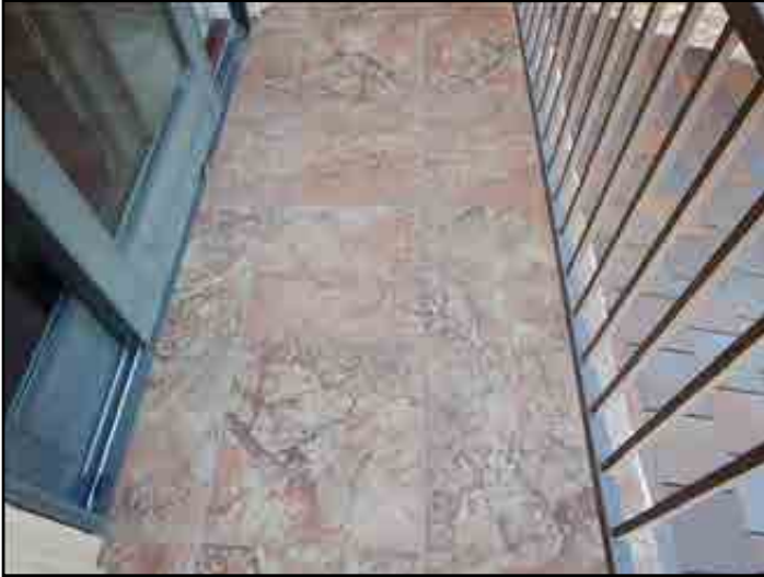
66. Cracked grout lines
