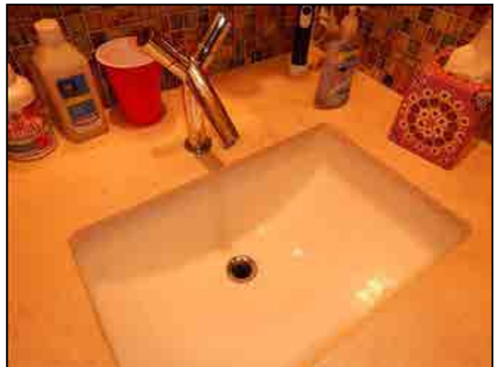
187. Drain stop missing
