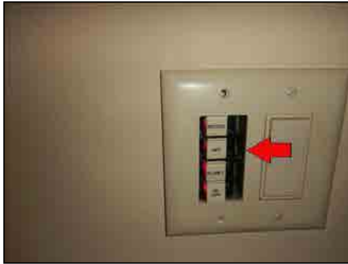
114. Damage cover plate
