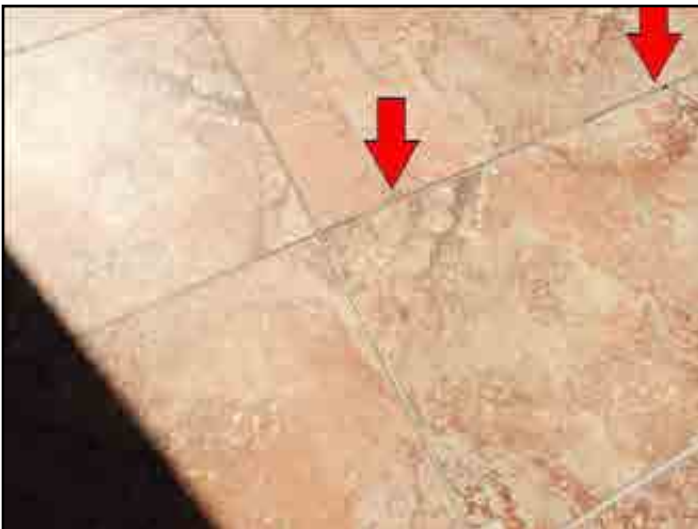
68. Cracked grout lines
