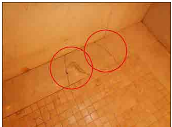
201. Tile loose, broken or missing tile
