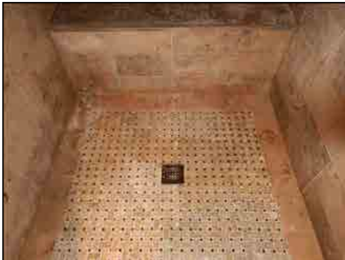
196. Caulking loose, missing or deteriorated
