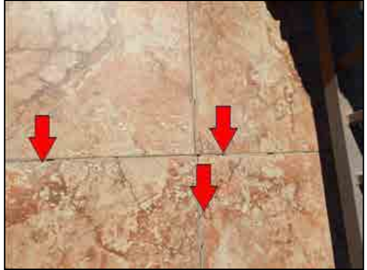
67. Cracked grout lines
