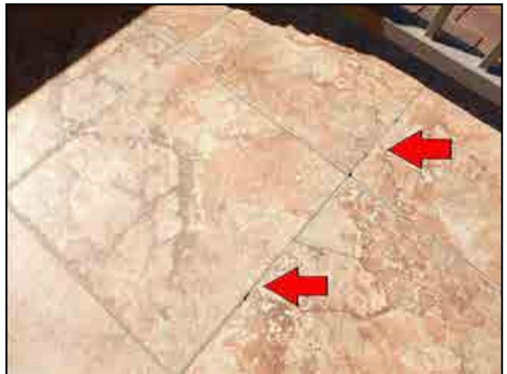
69. Cracked grout lines
