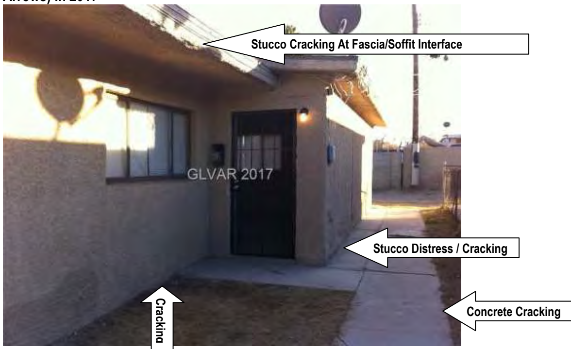
Photograph 2 (GLVAR-Supplied) Note Cracking/Distressed Stucco West Side And Cracked Concrete Slabwork (White Arrows) In 2017
