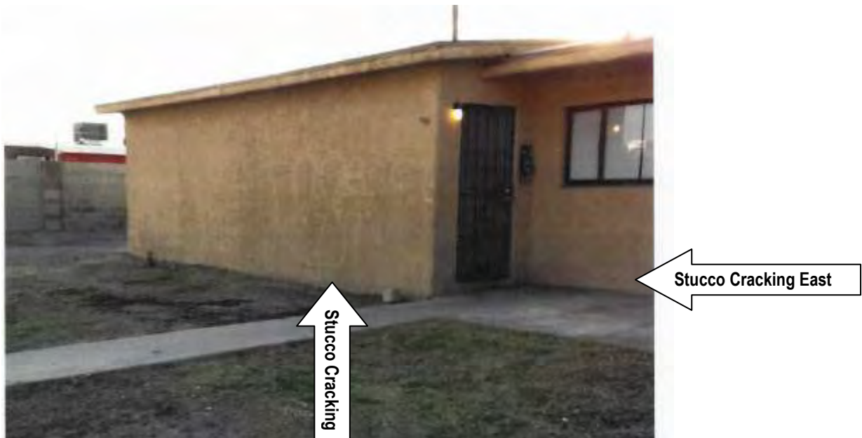
Photograph 4 Stucco Cracking At The East-Side Walls Of The Property (DEF 4000310)
