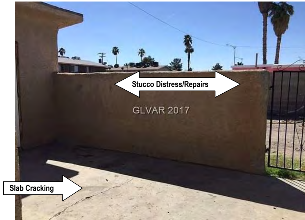
Photograph 3 (GLVAR-Supplied) Note Cracking/Distressed Stucco From South Patio Area On Wall And Cracked Concrete Slab (White Arrows) In 2017
