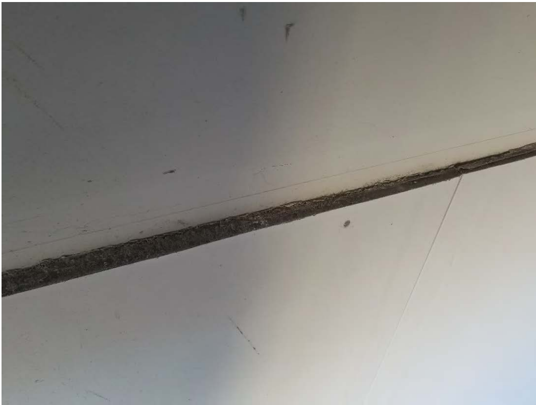
Top of Wallboard Right of C29-2 Sample – Dust Accumulation
