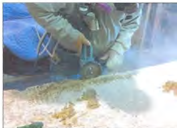
Cutting stone, as pictured, generates dangerous crystalline silica dust that can become trapped in lung tissue and cause silicosis.
