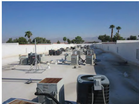
16. The flat roofs on the west side of the property consist of single-ply TPO membranes that are in good condition.
