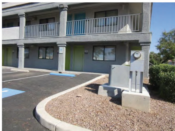
42. Pad-mounted electric transformers provide power to the buildings (note master meter).
