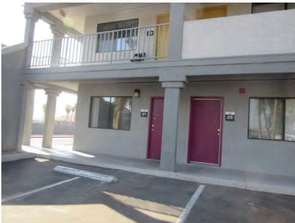
15. Building cladding includes painted stucco.
