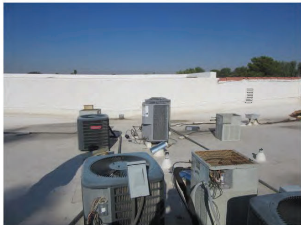
40. Approximately half of the condensers are over 20 years old.
