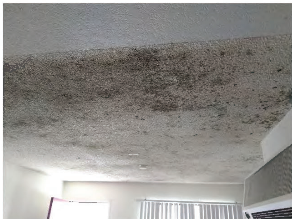
64. View of microbial growth in a down unit
