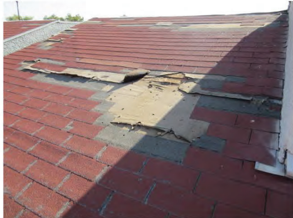
20. View of damaged composition asphalt shingled mansards.
