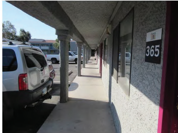
14. Building cladding includes painted stucco.
