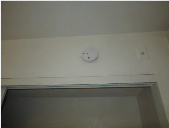
49. Hard-wired smoke detectors with battery back-up are mounted in each dwelling unit.
