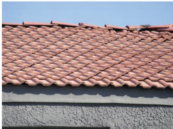
22. View of damaged concrete tiled mansards.
