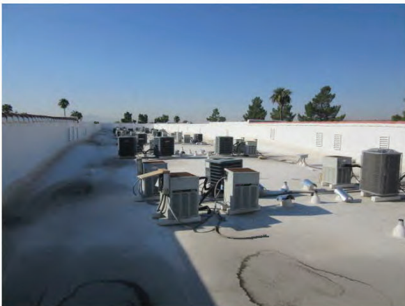
39. Cooling to the dwelling unit is provided by roof-mounted A/C condensers.
