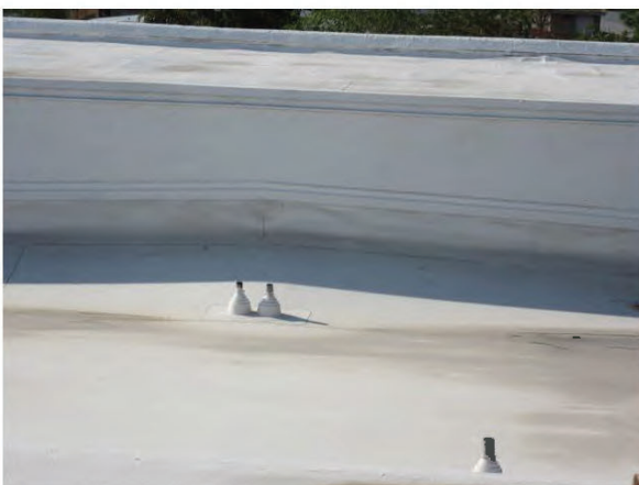
17. View of TPO roofing and flashing.
