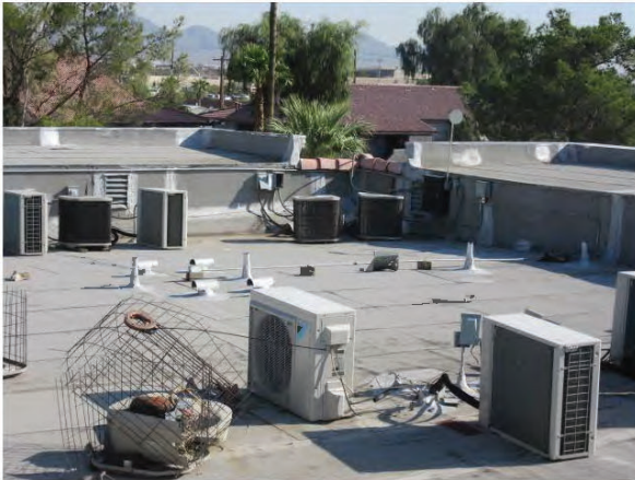
19. View of older modified bitumen roofing.
