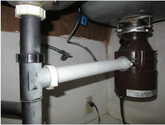
37. Drain lines are PVC.
