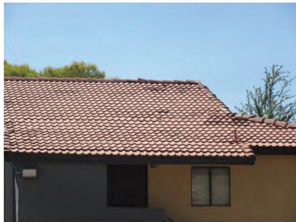
16. View of damaged concrete roof tiles.
