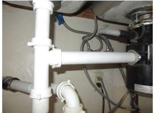
38. Drain lines are PVC.
