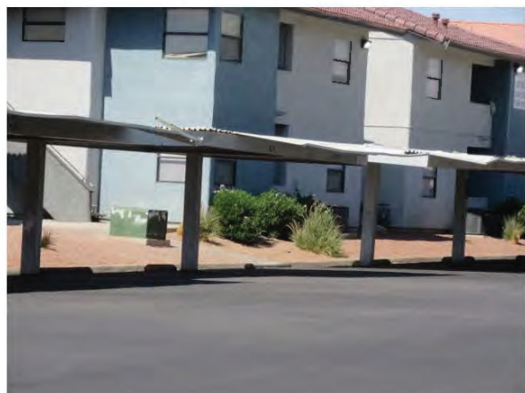
6. Steel-framed carports are installed throughout the Property parking area. Note vehicle damage to the roof.
