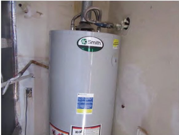
37. Domestic hot water is provided by individual natural gas-fired water heaters.
