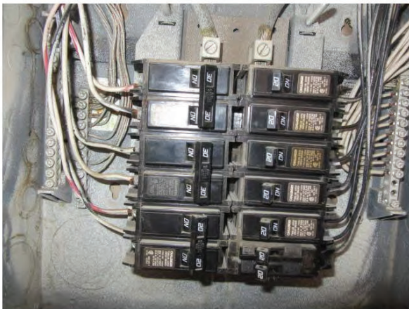
45. Branch wiring is copper.
