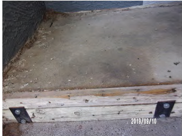
20. View of a water-damaged landing and missing carpet
