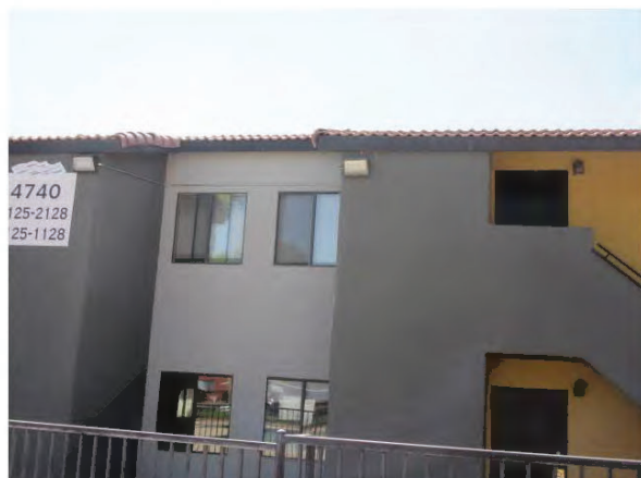
12. Building cladding includes painted stucco.
