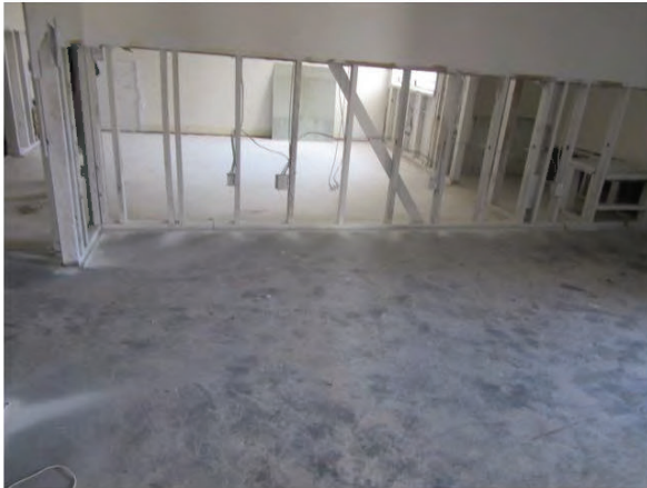
55. View of partially removed drywall and flooring in a down unit.
