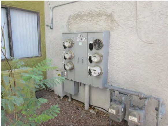
43. Electric service is individually metered.
