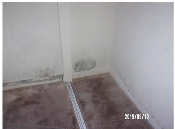
60. View of suspect mold growth in a down unit.
