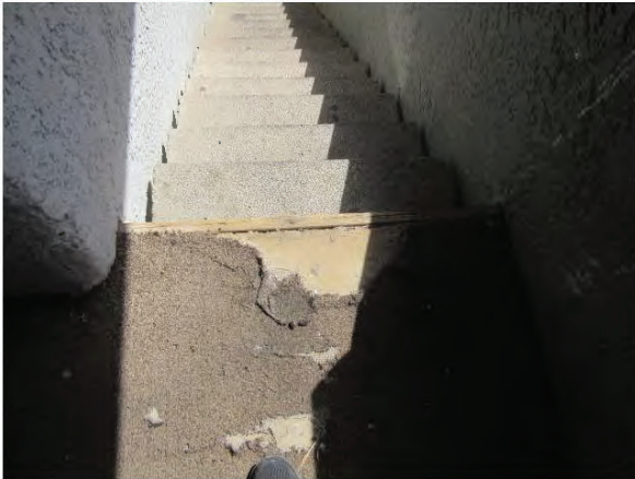
19. Elevated landings are plywood or OSB with outdoor carpeting. The landings are damaged.
