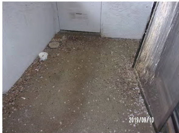
22. View of a typical patio/balcony with stained carpet from pigeon droppings.
