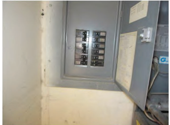
44. Breaker panels provide overload circuit protection.
