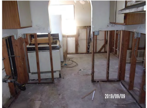
56. View of missing wallboard and flooring in a down unit.
