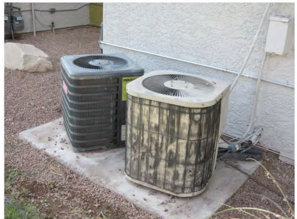
40. Cooling in the units is provided via pad-mounted A/C condensing units.
