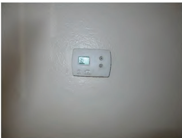
41. Temperature in the units is controls by manual wall-mounted thermostats.
