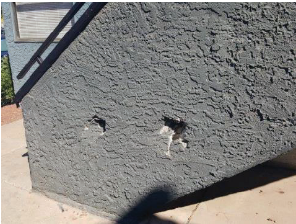
15. Punctured stucco covered stair system
