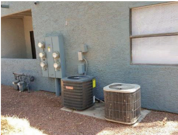
33. Pad mounted air conditioning condensers and main electrical switch gear and meters.
