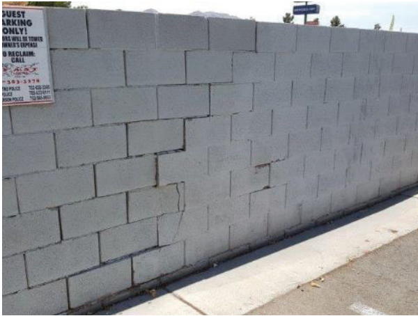
7. Damaged CMU perimeter wall
