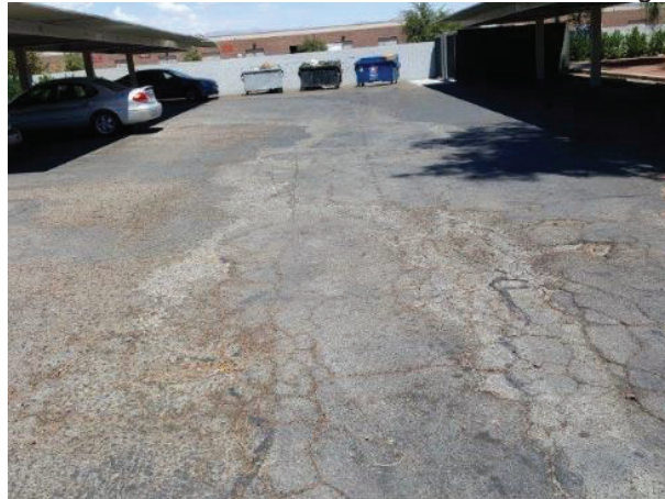
2. Severely damaged asphalt pavement
