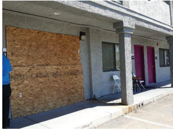
20. Unit 101's stucco cladded sidewall exhibited excessive vehicular damage. Reportedly a car drove into the stucco cladded sidewall. Plywood was observed over the window and sections of the wall.
