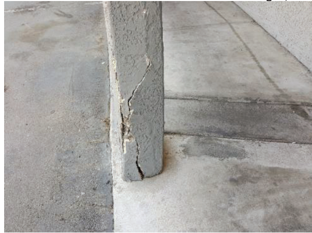
14. Stucco cladded columns were found cracked and severely damaged. This condition was observed near Unit 9 and 377.
