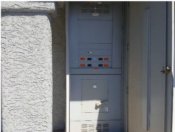
33. Each building is provided with a 600-amp, 240-volt service.
