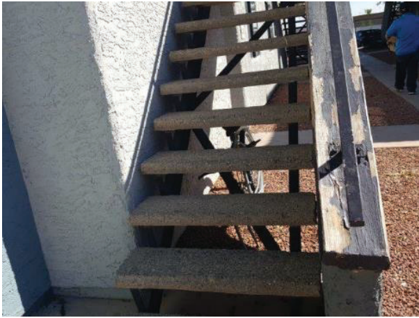
13. Dry rot on the wood handrail system
