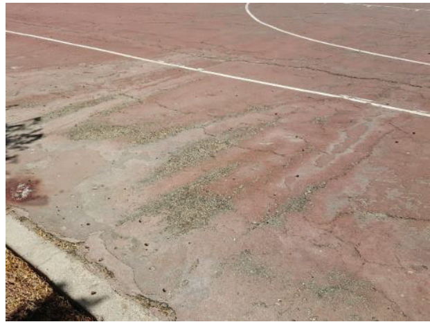
10. The basketball court exhibited surface deterioration and excessive cracks.
