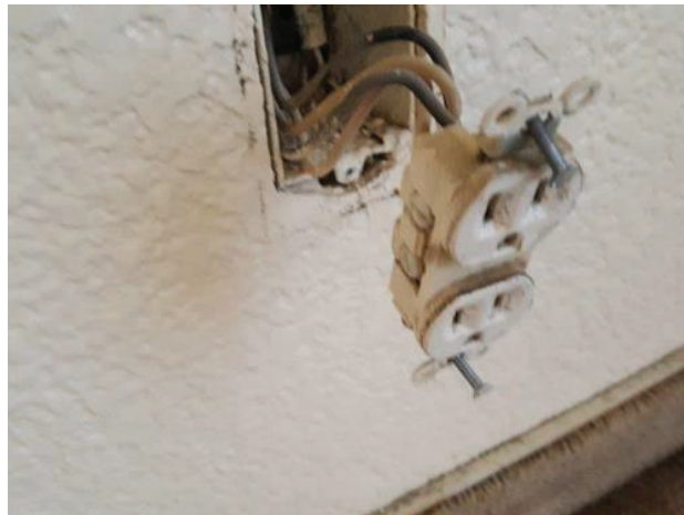
34. Open outlet verifying copper wiring
