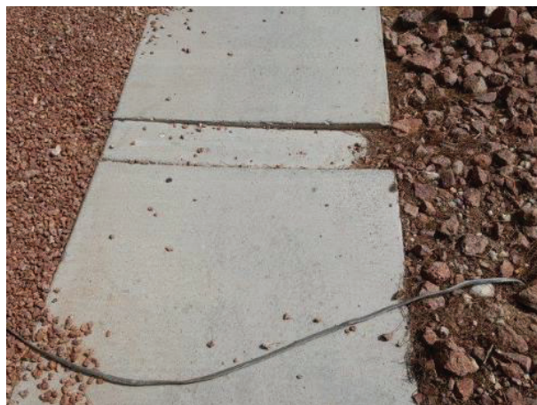
6. Uneven concrete sidewalk pavement (Repaired 10-17-2017)
