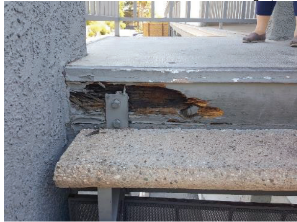
8. Stair systems exhibited excessive damage. Photographed above is an example of dry rot on wood the top risers. (repaired 10-7-2017)
