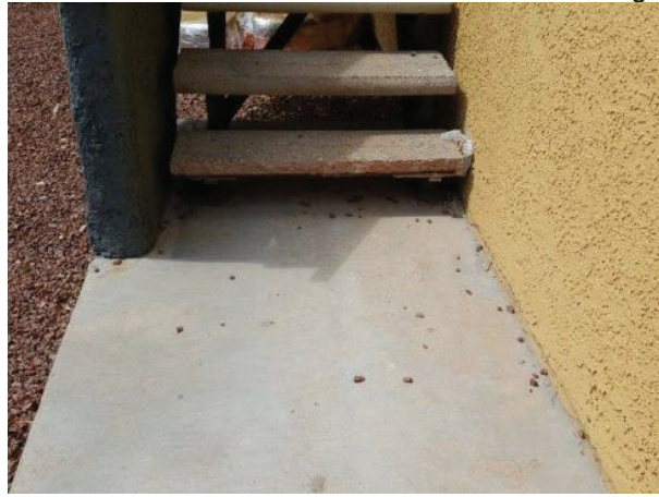
14. Broken concrete treads (repaired 10-9-2017)
