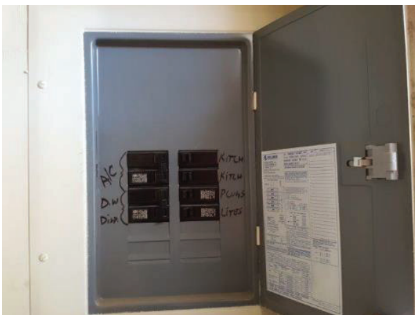
35. Circuit breaker located in each apartment unit
