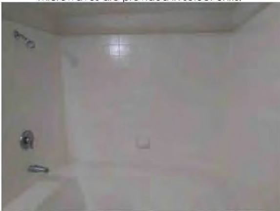
45. Bathrooms have a fiberglass tub with ceramic tile shower surround.
