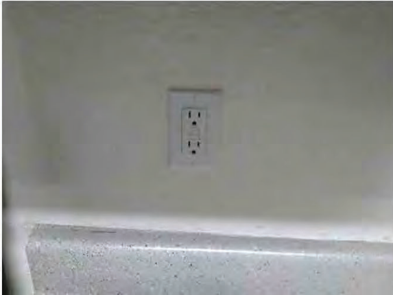
37. GFCI type receptacles were observed at unit wet areas (kitchens and bathrooms).
