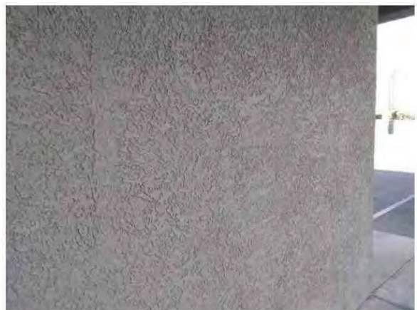
12. Typical painted stucco building exteriors.
