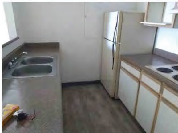
42. Kitchen cabinets are wood or laminated with plastic laminate countertops. Kitchen sinks are double bowl stainless steel.
