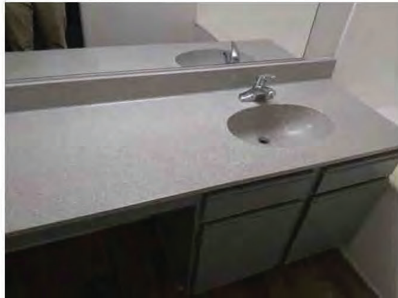
44. Bathroom vanities are wood with cultured marble counters and integral sinks.
