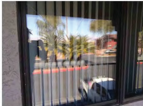
22. Building windows are double-pane sliding units in metal frames.
