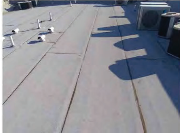
14. Typical modified bitumen roofing.
