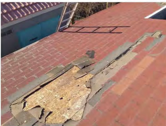
17. View of damaged composition asphalt shingled mansards.
