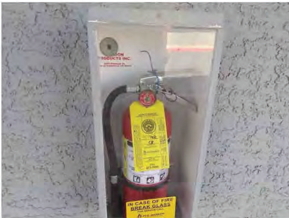
39. Fire extinguishers are mounted at common areas. Inspection tags are current.
