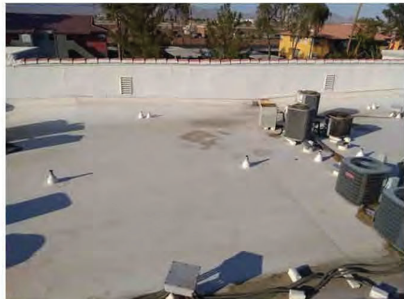
16. Typical TPO membrane roofing.
