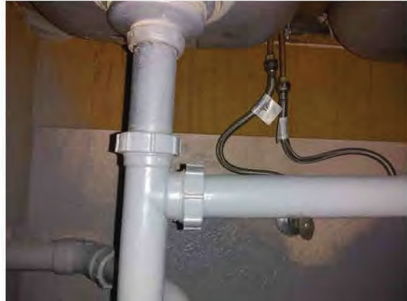
32. Building drain lines are PVC.
