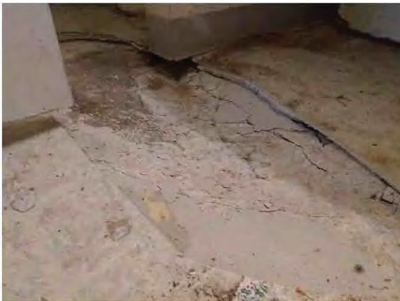
51. View of damaged floor in down unit 136.
