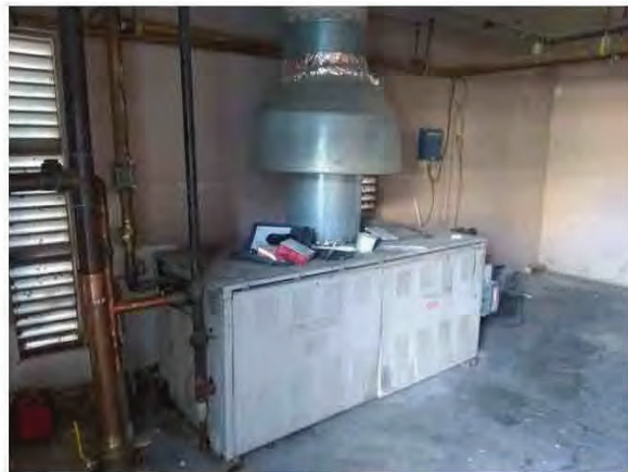
30. Heated domestic water is provided by domestic boilers and storage tanks. Building supply lines are copper.
