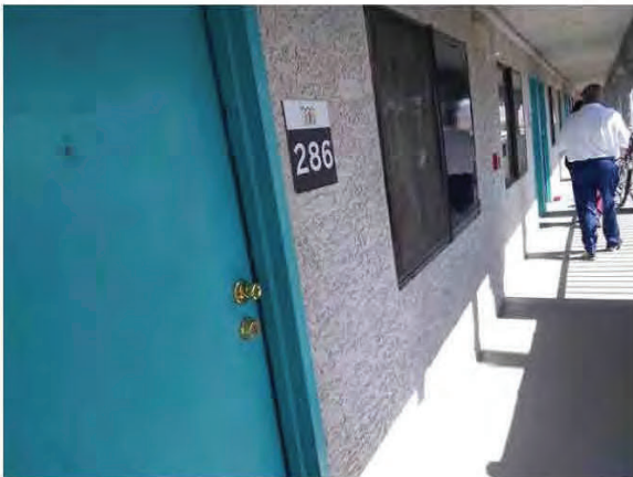
21. Typical upper level walkway. Unit entry doors are wood assemblies in wood frames.
