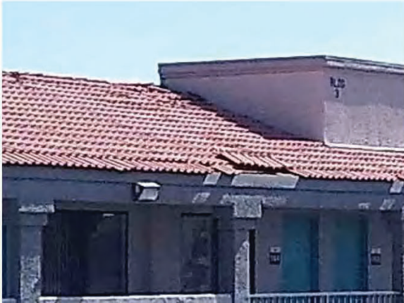
19. View of damaged concrete tiled mansards.
