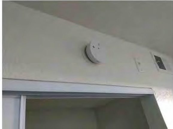
38. Hard-wired smoke detectors with battery back-up are mounted in each dwelling unit.
