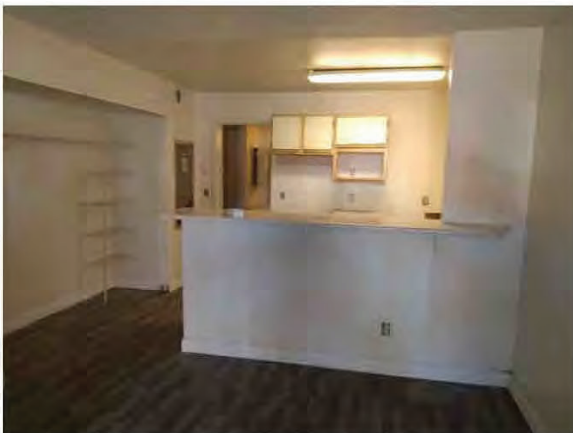
41. Dwelling units have painted drywall walls and ceilings. Vinyl floor tile is installed at select unit living areas and bathrooms.
