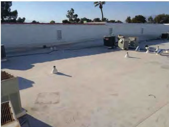
15. The flat roofs on the west side of the Property consist of single-ply TPO membranes.
