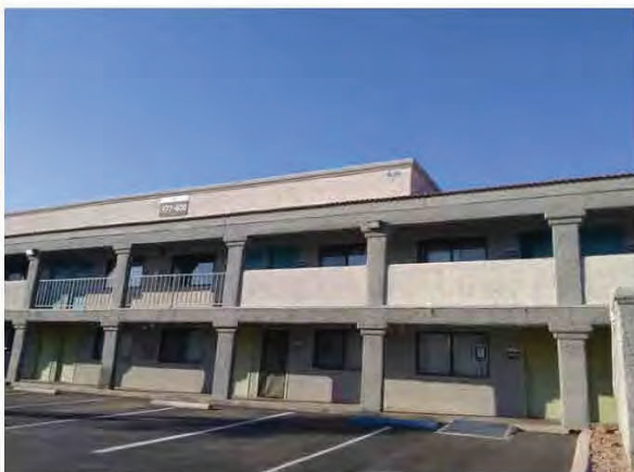
11. Building cladding includes painted stucco.
