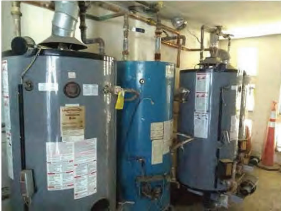
31. Central natural gas-fired water heaters also provide domestic hot water to the Property.
