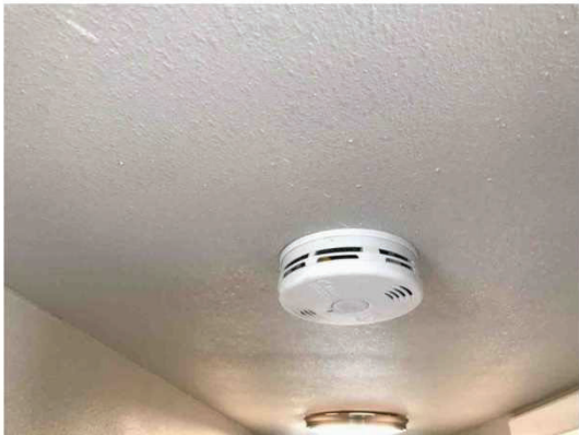
Smoke Alarm/Carbon Monoxide Detector
