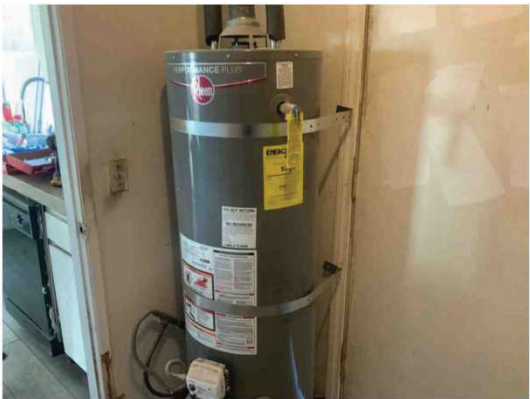
Water Heater Double Strapped
